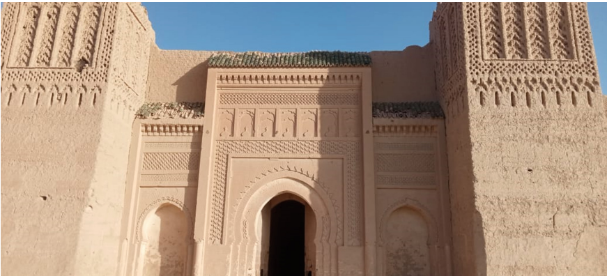
Fig. 2. The main entrance to ksar abbar in rissani
