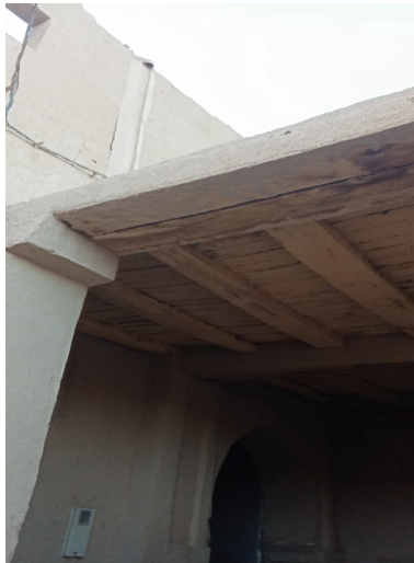
Fig. 5. Wooden roof
