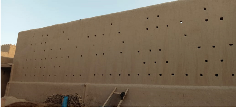
Fig. 3. Rammed earth wall
