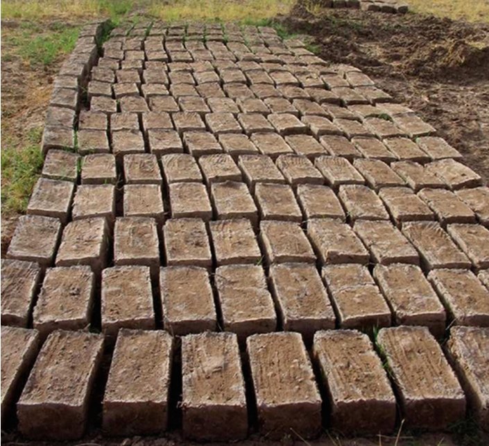
Fig. 4. Mud brick sun dried. Credit by Baglioni [5]
