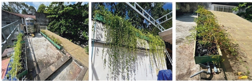
Fig. 7.5 Green roof systems at Ho Chi Minh University of Technology
