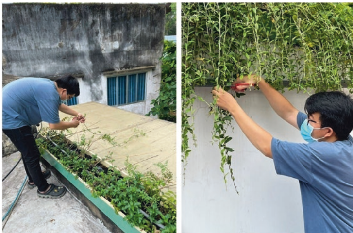
Fig. 7.6 Taking care and pruning the green roof system
