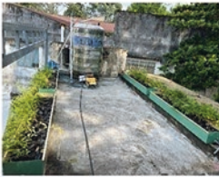
Step 7. Adding plants in the green roof system.
