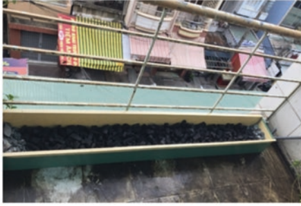
Before the installation
