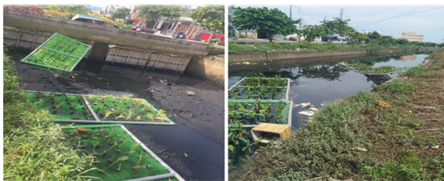
Fig. 10.15 Some common problems
