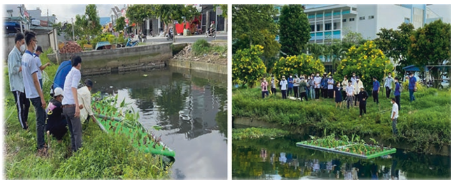
Fig. 10.12 Launching and fixing the rafts
