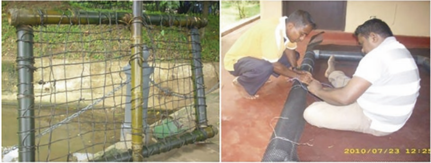
Fig. 8.13 Preparation of rafts by both Bamboo and PVC
