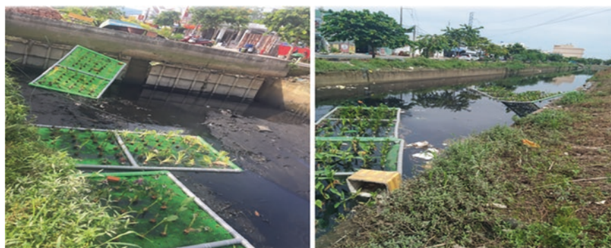
Fig. 10.15 Some common problems
