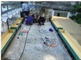
Step 3. Installation of the tray, pump, pipe, and electrical systems
