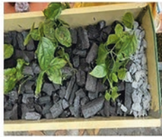
Step 7. Adding plants in the green roof system.
