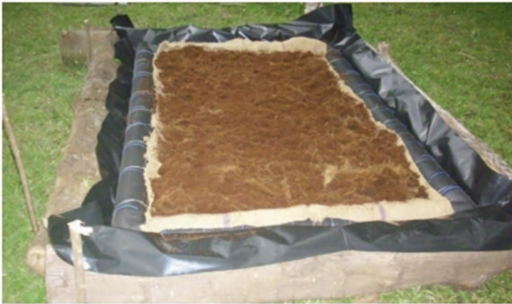
Fig. 8.14 Introducing coconut coir to the constructed rafts
