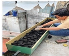
Step 5. Adding charcoal on top of the oyster shell layer
