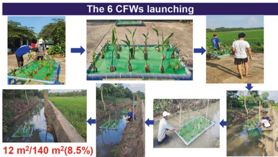
Fig. 11.2 The installation and launch of six CFWs
