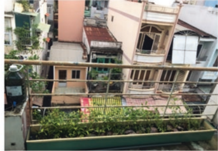
After completing the installation
