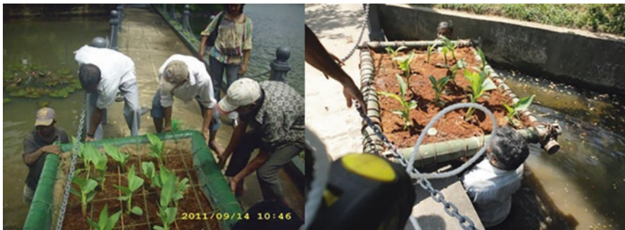
Fig. 8.18 Maintenance and implementation of CFWs in Kandy Lake, Sri Lanka
