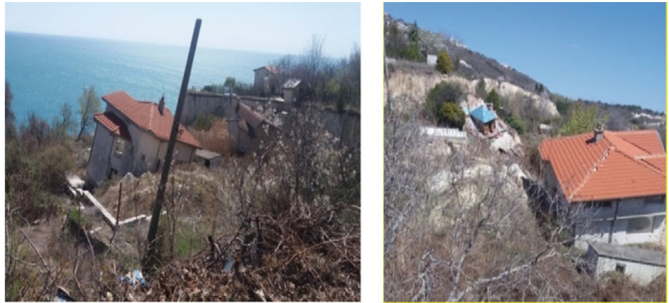
Fig. 1 Recent developments of Fish-Fish landslide (photograph taken by authors in April 2019)
