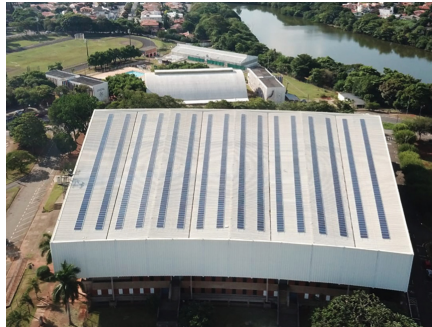
Fig. 1. Photovoltaic Energy Plant of the UNICAMP Multidisciplinary Gymnasium (GMU-PV).
