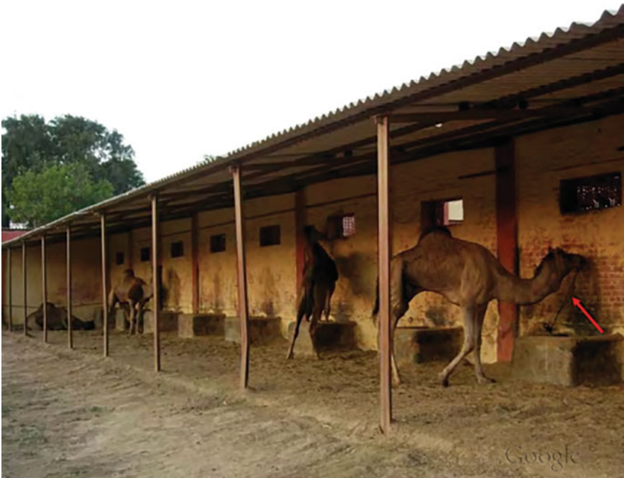
Fig. 5.12 Asbestos-roofed open-type shelter with an animal tied on the individual manger
