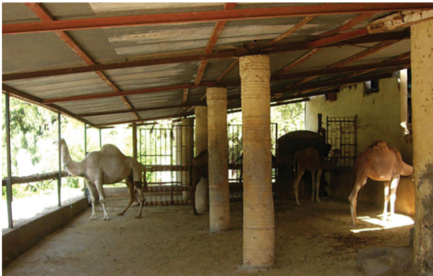
Fig. 5.8 Asbestos-roofed open-type shelter
