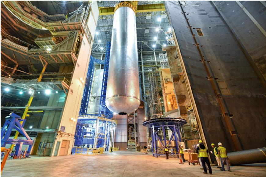
Fig. 2 Boeing technicians move the SLS EM1 LH2 hydrogen tank. NASA/Steven Seipel under CC0 1.0 Universal
