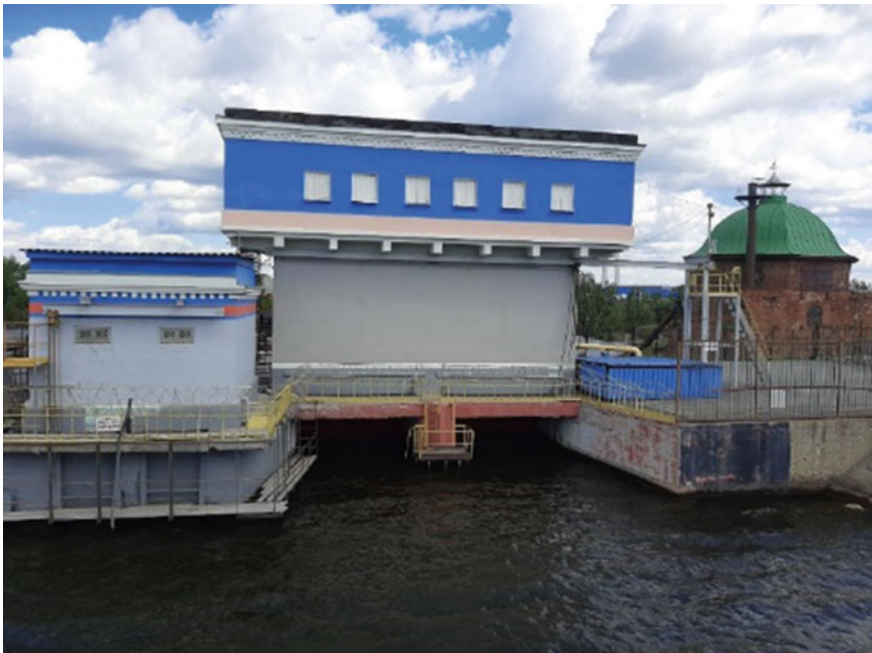
Fig. 6 The dam of the Seversky plant. Polevskoy. Photo by V. Litovski. 2022
