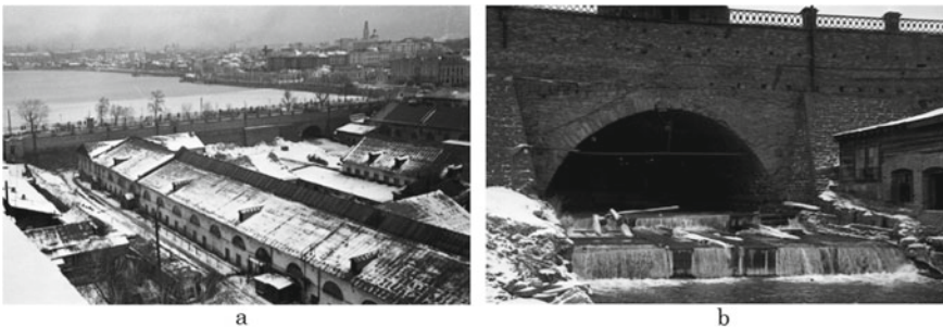
Fig. 2 a Production buildings at Plotinka before the start of work on the creation of the historical square. Sverdlovsk. Early 1970s GASO (State archives of the Sverdlovsk region). F-1. Op. 6. D. 6376; b Dam before reconstruction. Sverdlovsk. Early 1970s GASO. F-1. Op. 6. D. 6388
