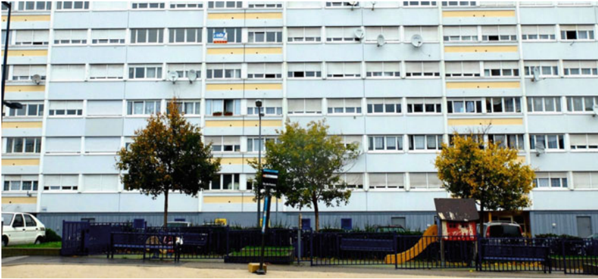
Fig. 2 An example of the renovation of a high-rise building in France under the national urban renewal program
