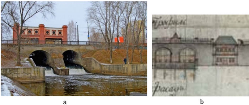
Fig. 5 a Nizhne-Isetskaya dam. Ekaterinburg. Modern look. Photo. Source The first bulb of Nizhneisetsk. Museum of Energy of the Urals. URL: http://musen.ru/chronicle/1921/ ; b “Profile plan and facade of the Nizhne-Isetsy state-owned plant to the dam, rebuilt according to the design of the Ekaterinburg Mint by the foreman Egor Usoltsev”. GASO. F. 25. Op. 2. D. 7927. Source 14, p. 11. Fragment
