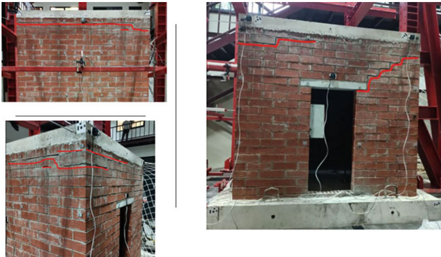
Fig. 5.4 The pattern of damage on the specimen's external surface for the DS-4 type
