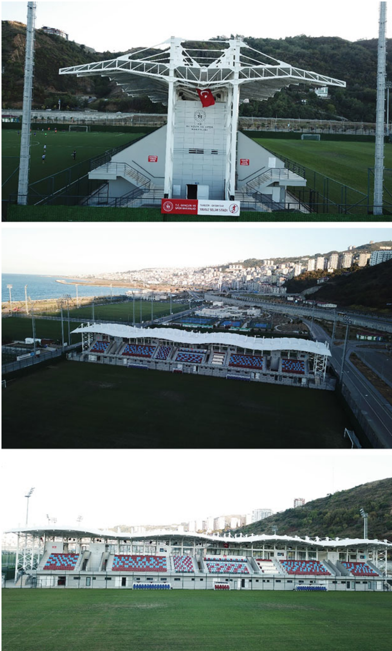
Fig. 10.6 Pictures after the completion of the tribune project
