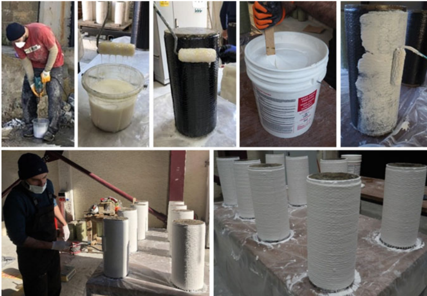
Fig. 9.2 Preparation and application of the System B components
