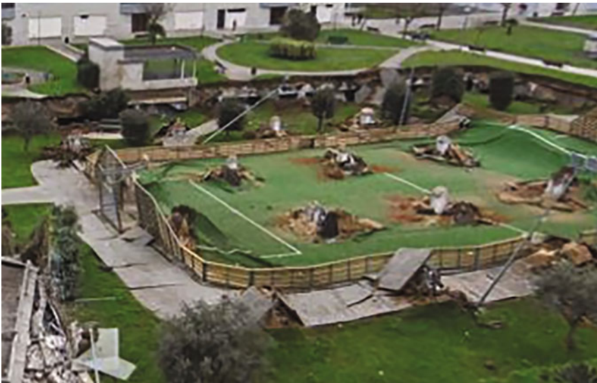
Fig. 14.1 Parking garage atop a playground collapsed (Deifalla 2022)
