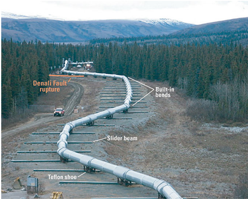
Fig. 11.4 Alaska pipeline crossing at Denali Fault ( Source US Geological Survey)
