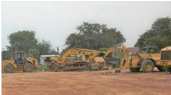
Fig. 6 Some earthmoving equipment in central workshop awaiting repair
