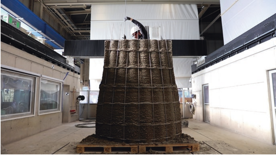
Fig. 3 Threading unbent vertical reinforcement into the shotcrete core structure. (Image courtesy Norman Hack)
