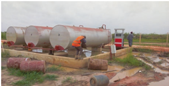
Fig. 3 Fuel depot at field workshop to ease fuel supply to machines right on the field
