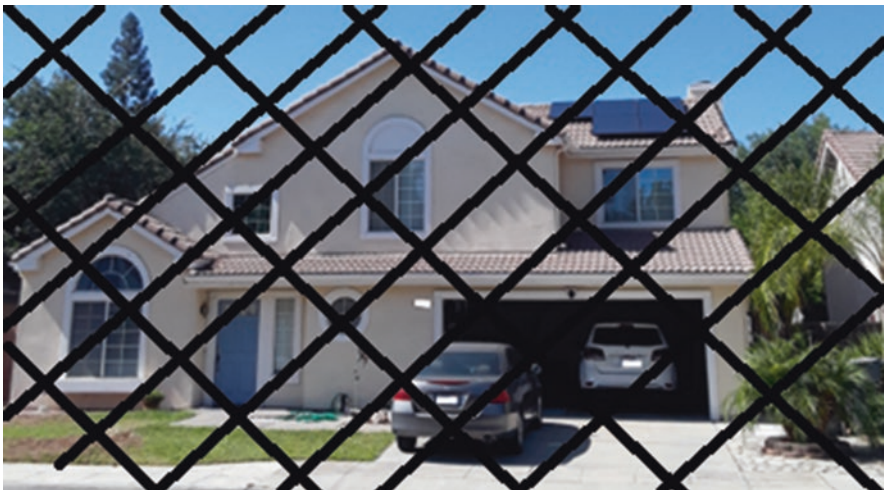
Fig. 5 A smart home that has zero electric bill and is good for 25–30 years. [Note: for the purpose of security, the image has been made such]
