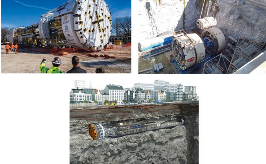
Fig. 2 Tunnel-boring machine (TBM)
