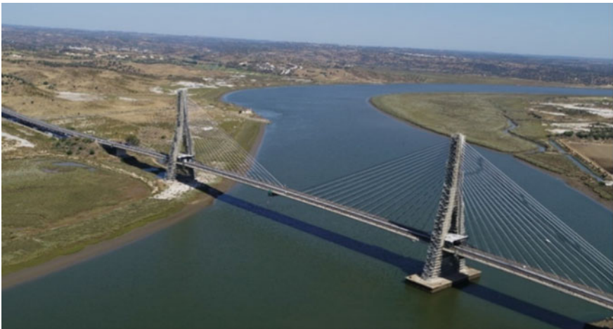
Fig. 1 Aerial view of Gadiana International Bridge during stay cable replacement works [4]
