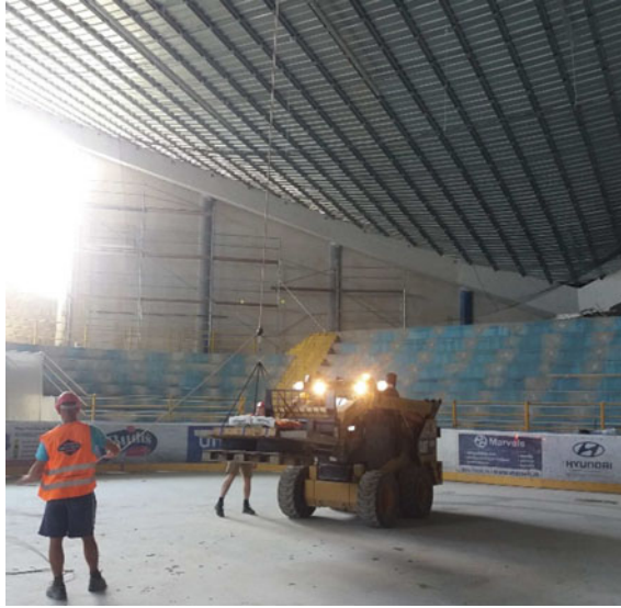
Fig. 5 View of the hanging mass before release
