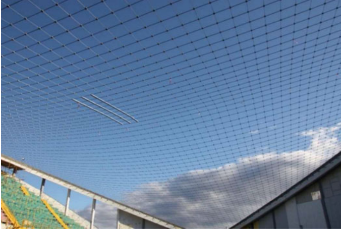
Fig. 3 View of the cable net from inside the structure
