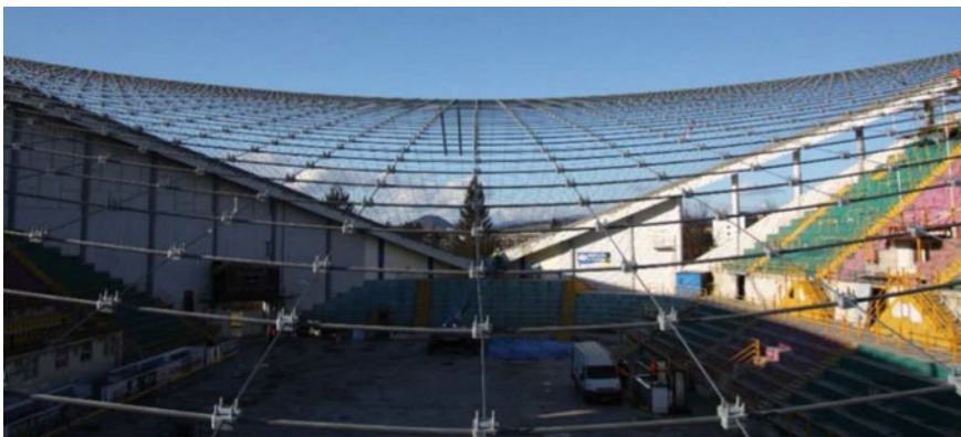
Fig. 2 Side view of the cable net
