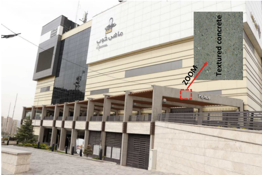
Fig. 2. Textured concrete performed by the construction company of Gohar Sang Gareh Dag (Tabriz, Iran)
