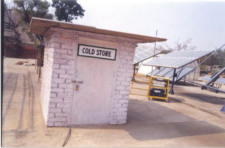
Fig.24 Solar photovoltaic powered cold store (Eltawil and Samuel 2007b)
