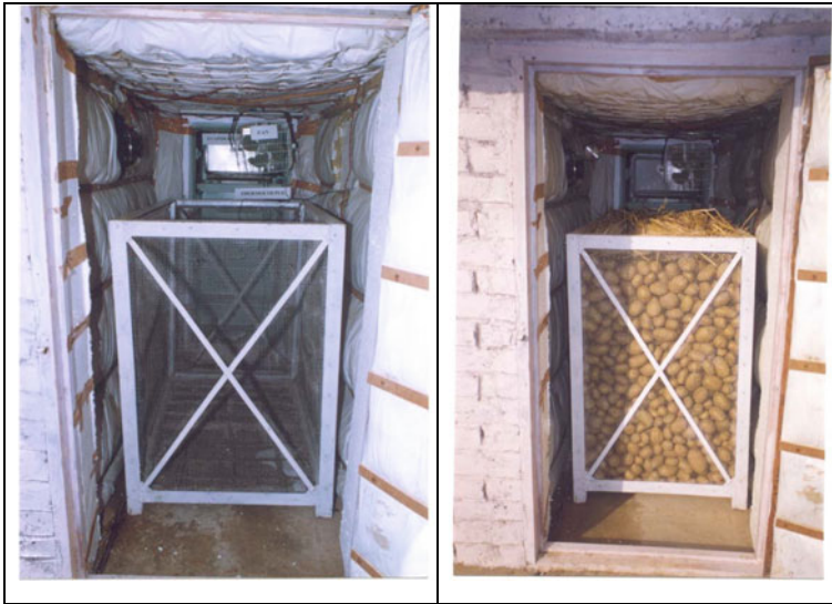
Fig. 26 Inside view of cold store structure without load and loaded with cured potato tubers (Eltawil 2012)
