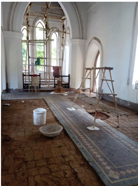
Fig. 6 Original 19th-century tile flooring revealed when the later additions were carefully removed during the conservation process. Source Second author, adapt
