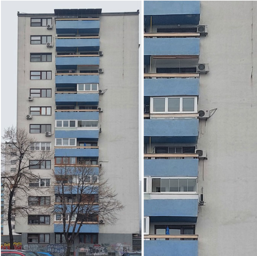
Fig. 4 Exterior air conditioners on the skyscraper façade
