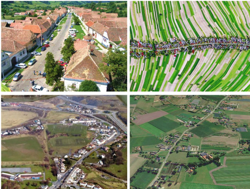
Fig. 3 Villages Valea Valor, Romania and Suloszowa, Poland, (up) and ribbon developments near Merthyr Tydfil, Wales and near Limburg, Belgium (down) (Sources Websites; valea-viilor.ro , World Urban Planning IG, ggaat.org.uk , google satellite image)
