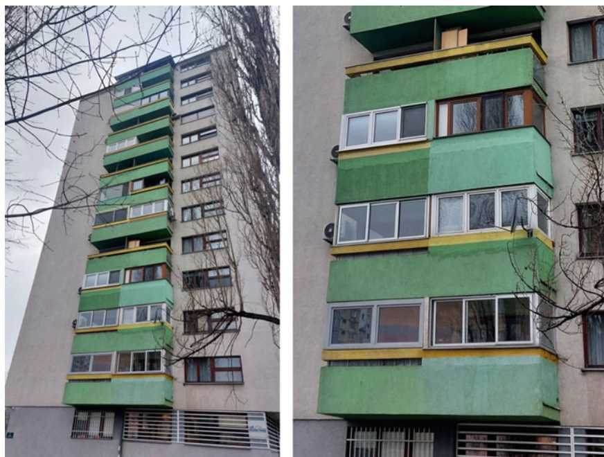
Fig. 3 Different approach and realization of glazed balconies on the façade of a skyscraper
