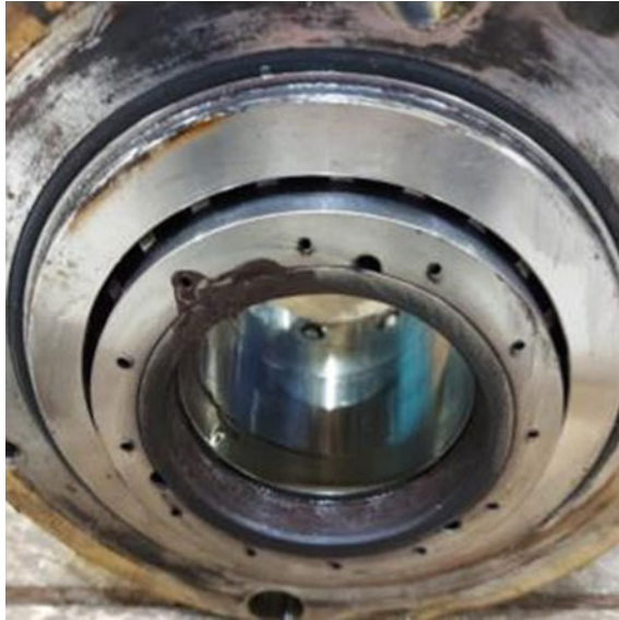
Fig. 8 A thermal stress and hot spot on bearing housing
