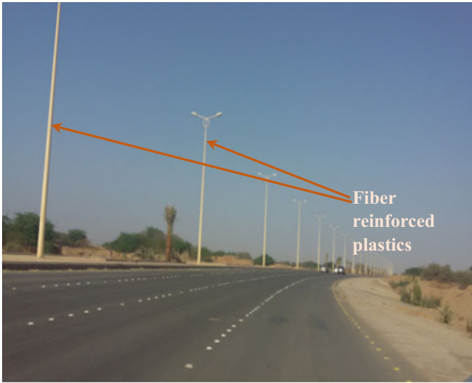
Fig. 1 Light poles made of FRPs
