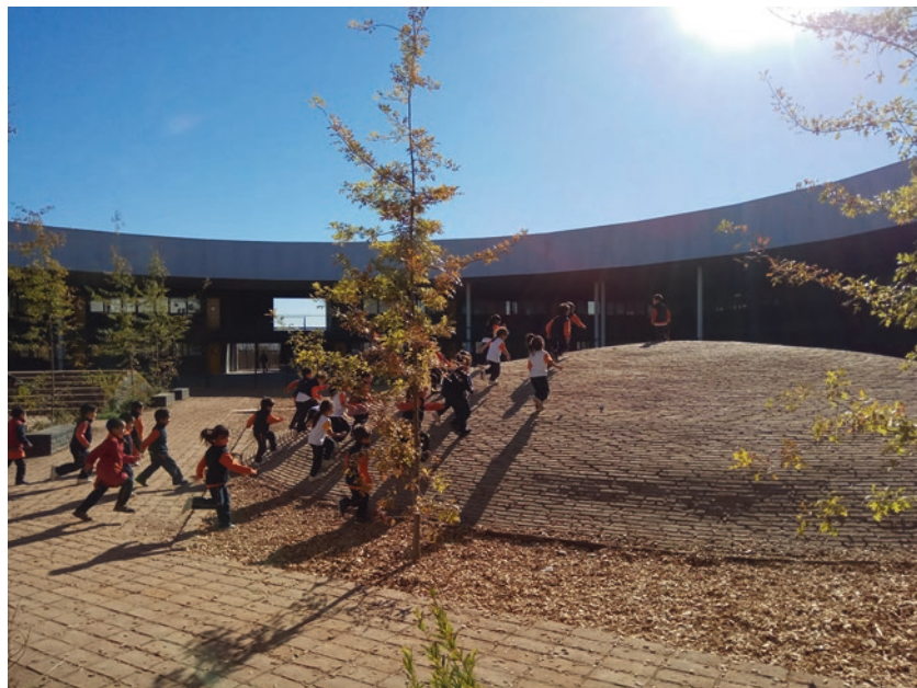
Image 35.3 Brick hill for free play in Aylén School. (Credits: Patio Vivo Foundation)
