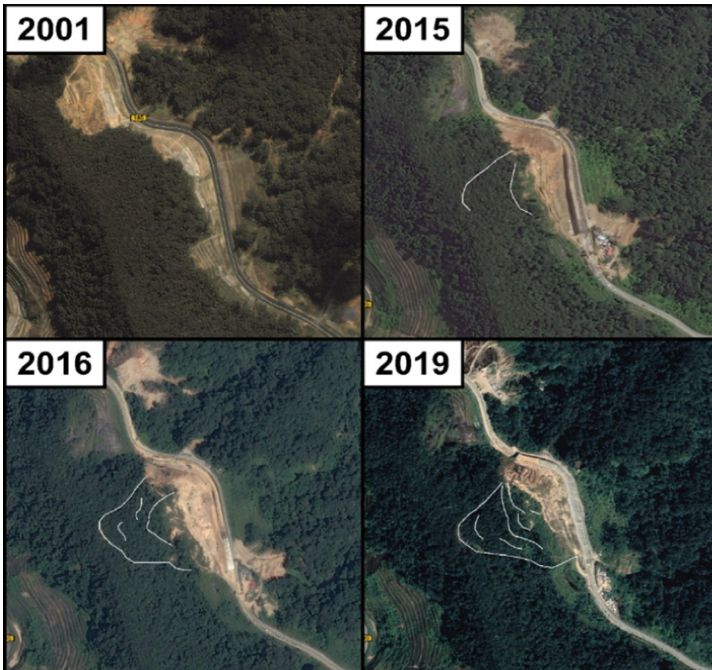
Fig. 6. Trend in tension cracks of Gunung Pass from year 2001 to 2019.
