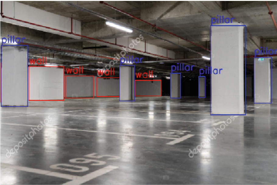
Fig. 5. Annotated Image of Indoor Parking Lot.
