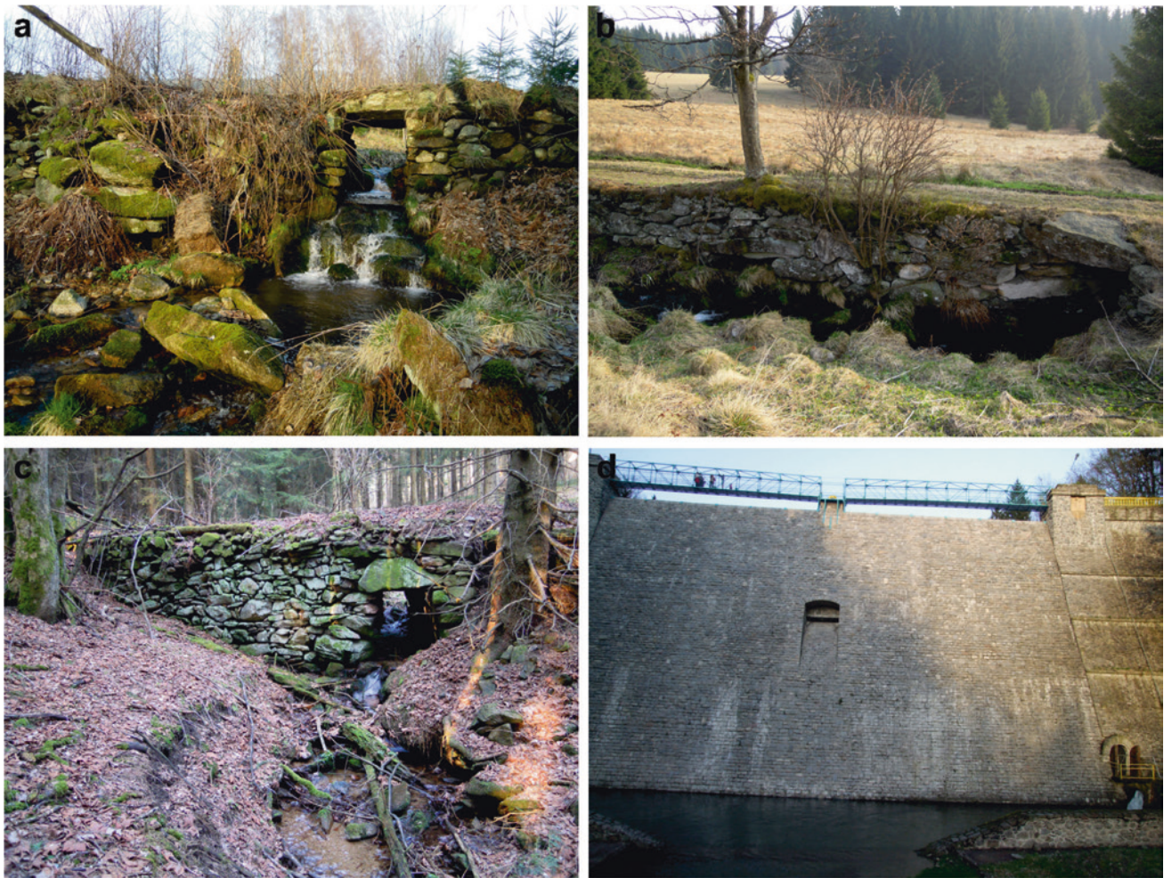
Fig. 11.7 Diversity of water management constructions; examples. a Stone bridge. b River bank reinforcement. c Check dam (all examples from the upper reach of the Nysa Kłodzka river). d Dry flood
