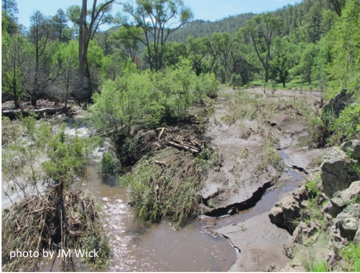
Fig. 10 Debris and fine sediment deposits in Black Canyon in Barrier-Private reach following the 2013 Silver Fire
