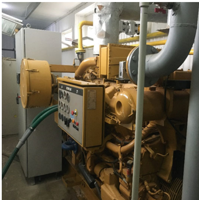
Fig. 23 Landfill gas to power generator on the base of a Caterpillar G3508 engine with electric power 500 kW
