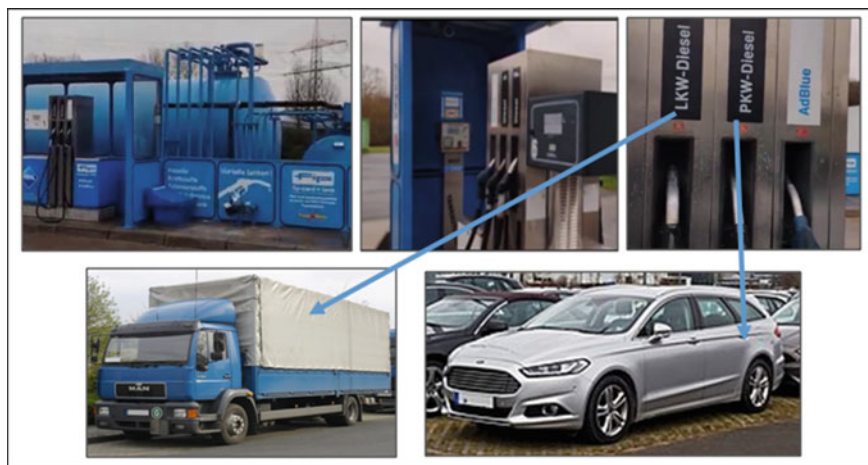
Fig. 3 Distribution complex at a gas station for the sale of diesel fuel and AdBlue reagent in Germany (photo August 2022)
