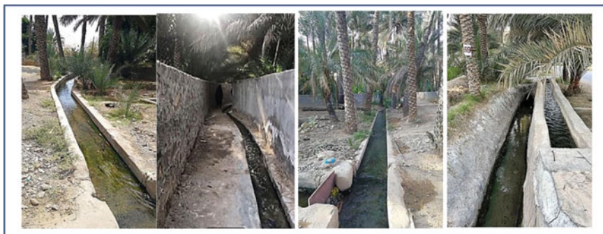
Fig. 16.1 A general view of water channelization through falaj in different regions in Oman. (Pic courtesy: Mohd. Taleb Sulaiman Al Shaqsi, Taif Rashed and Arwa Khamis Juma Al Dawdi)
