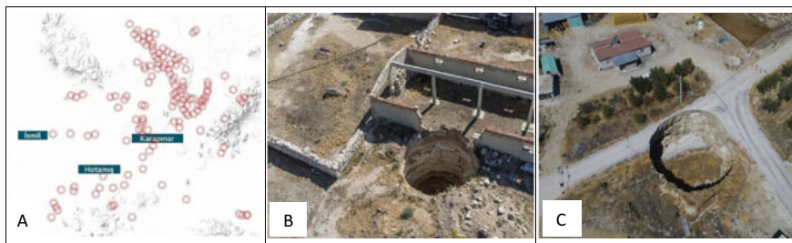
Fig. 11 Sinkholes in Konya a Sinkhole locations [6], b Konya [36], c Karapınar, Konya [18]
