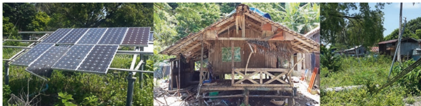
Fig. 5.4 Climate change impacts on technical equipment. Solar panels destroyed by hail and storm ( left ), house destroyed by a storm ( middle ), electricity lines destroyed ( right ), Bulon Don island, Thailand. (Taken by Katrin Lammers, 2017)
