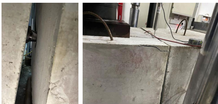
Fig. 5.11 Failure mode of shearing tests
