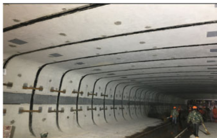
Fig. 4.17 Application of two-half-assembled precast concrete tube in RPJM
