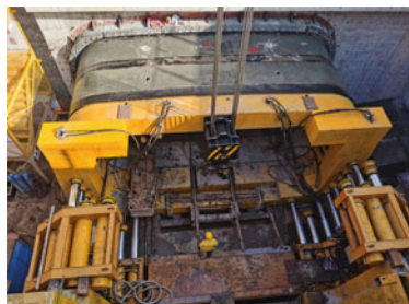
Fig. 4.17 Application of two-half-assembled precast concrete tube in RPJM
