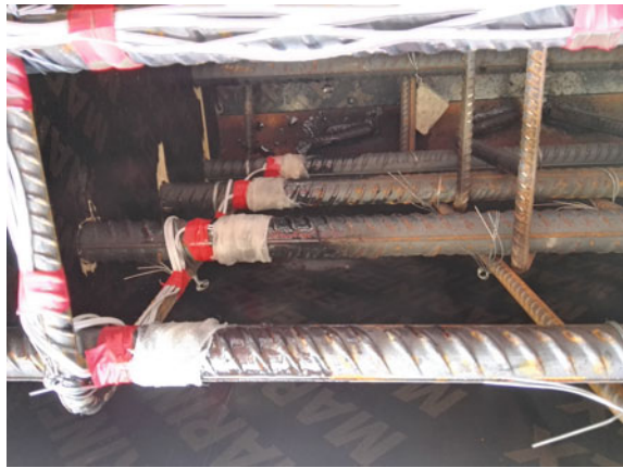
Fig. 4.7 Picture of measuring points of steel bar
