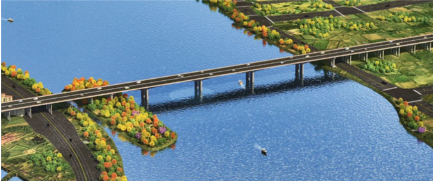
Fig. 39.1 Aerial view of the Nanyang Xiangjiang bridge
