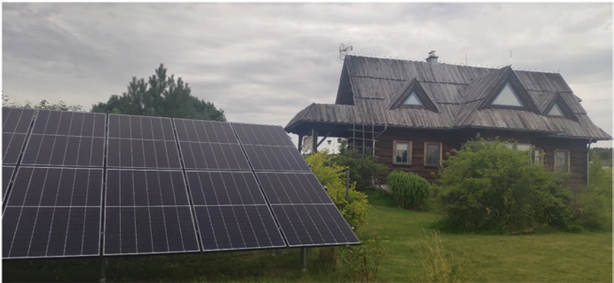
Fig. 9 PV modules settled on the ground as detached structures
