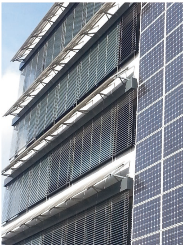
Fig. 13 BIPV – Building Integrated PV systems as cladding and solar shading devices
