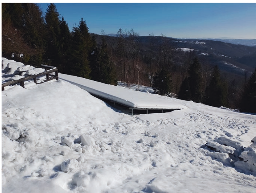
Fig. 12 PV system located on a small slope of the hill in January in Polish mountains
