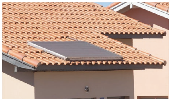
Fig. 3 Example of PV household installation as part of Luz para Todos for home without access to electricity
