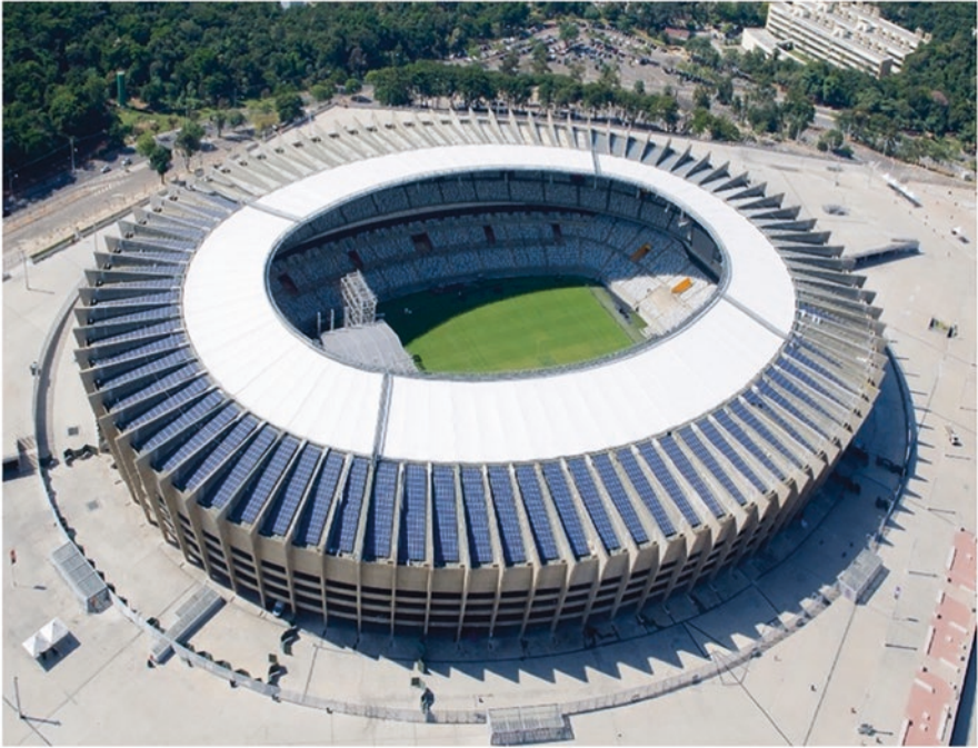
Fig. 22 Mineirão Stadium in Belo Horizonte, Brazil (1.3 MW crystalline-Si PV). One of four Brazil football stadiums integrated with PV for the 2014 World Cup
