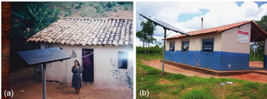
Fig. 2 Typical PV-electrified buildings through the (a) Luz Solar (single-family rural household); and (b) Luz no Saber programs (school). The PV was in these cases was not applied on the room in order to ensure security, structural integrity, and safety. Some homes did also have the PV systems roof-mounted if these three criteria were satisfied
