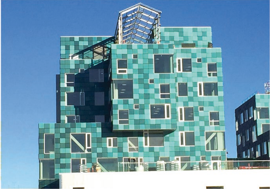
Fig. 10 Side view of the blue-green coloured Glass PV panels of Copenhagen International School in Nordhavn, Copenhagen, Denmark. (Image credit and source: Jens Cederskjold from København S, Denmark, https://actu.epfl.ch/news/the-school-with-the-largest-solar-facade-in-the%2D%2D9/ )
