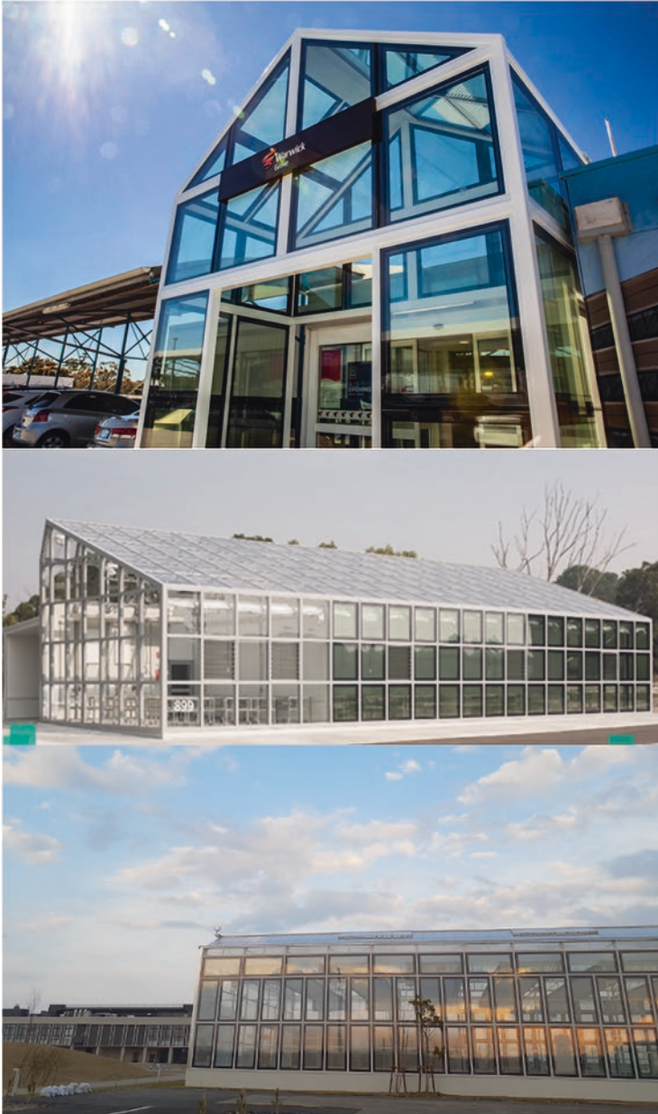
Fig. 1 High-transparency ClearVue solar windows deployed in commercial property-based and agricultural R&D and production facilities. Top: shopping centre atrium incorporating PV windows installed in 2019 in Perth, Australia; Middle: solar glazing-based greenhouse installation (2021) at Murdoch University (Perth, Australia); Bottom: wall of solar windows installed at a commercial greenhouse built in Sendai, Japan. (Image reproduced from Tomita Technologies website, 2022)
