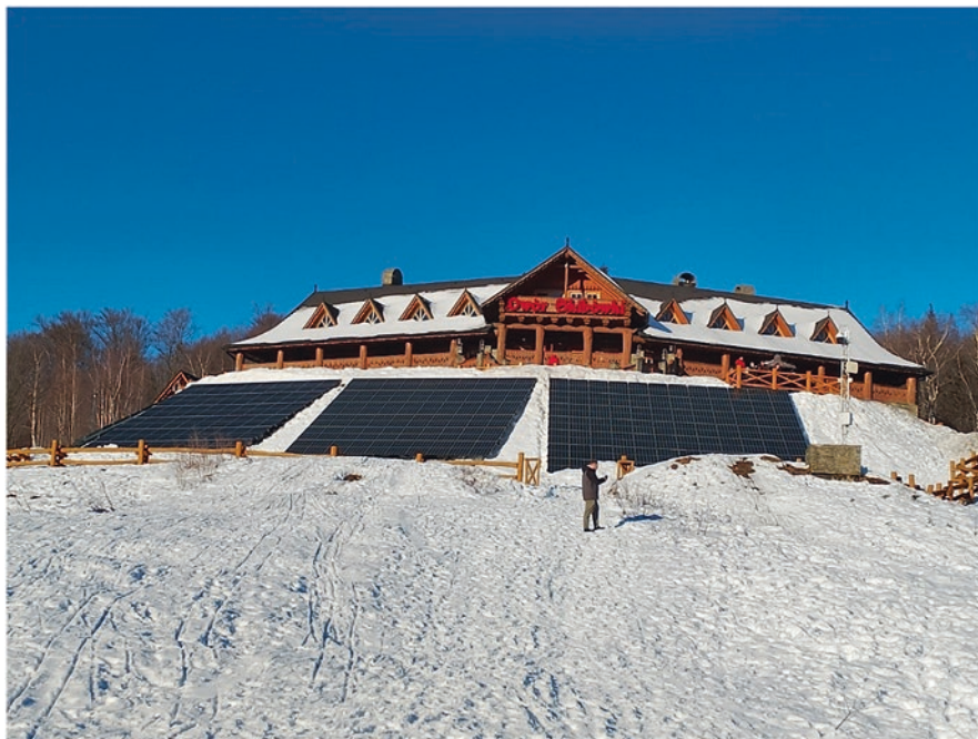
Fig. 11 PV system located on a high slope of the hill in January in Polish mountains
