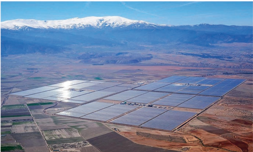
Fig. 31 Andasol Solar Concentrated Power Station (150 MW) near Guadix in Granada, Spain. (Image credit and source: Kallema, https://commons.m.wikimedia.org/wiki/File:Andasol_Guadix_4.jpg )
