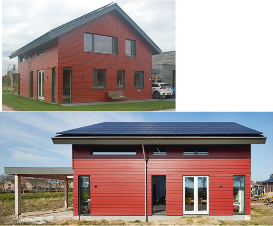
Fig. 15 BIPV roof of the House of Tomorrow Today 2.0
