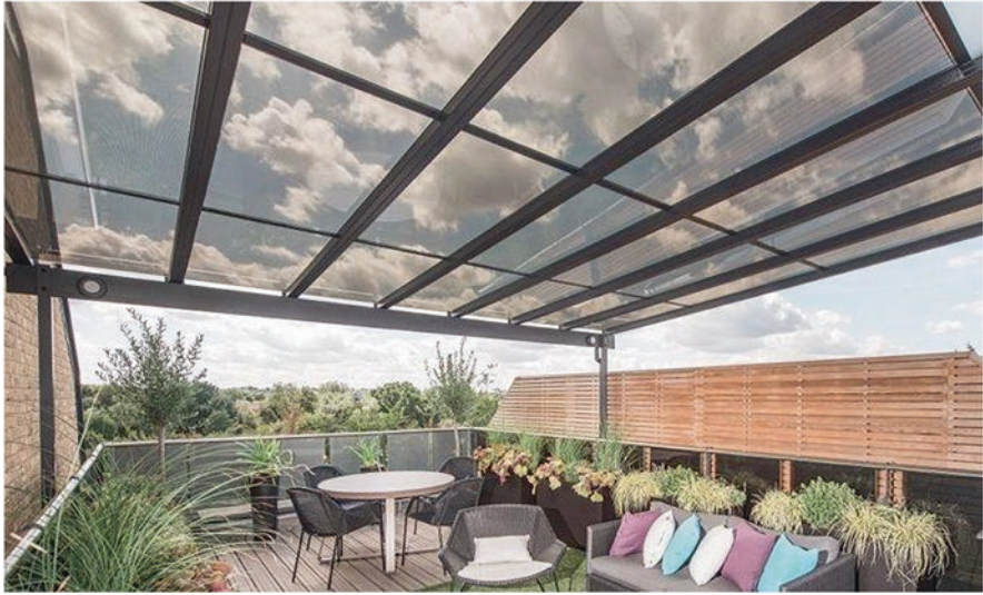
Fig. 5 Architectural solar glass – PV canopy, https://www.polusolar.co.uk , [8]
