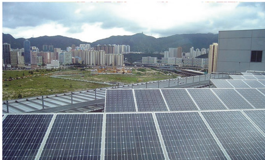
Fig. 19 Mounted solar photovoltaic arrays on rooftop of Electrical and Mechanical Services Department Headquarters' Photovoltaics in Hong Kong, China. (Image source: WiNG, https://commons.m.wikimedia.org/wiki/File:Electrical_and_Mechanical_Services_Department_Headquarters_Photovoltaics.jpg )
