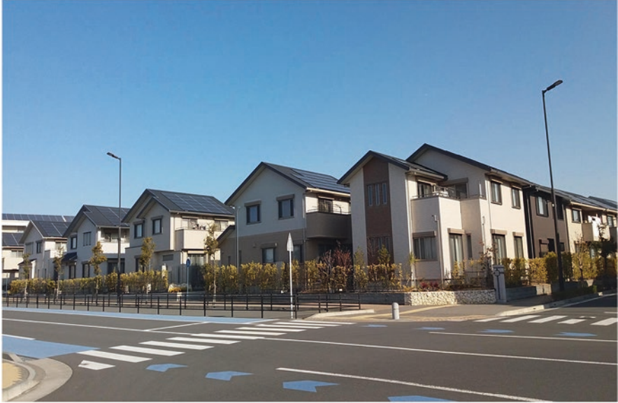
Fig. 35 Part of solar high-efficiency PV array installed at the fence of Fujisawa smart City in Yokohama, Greater Tokyo, Japan. (Image credit and source: Mohsen Aboulnaga)
