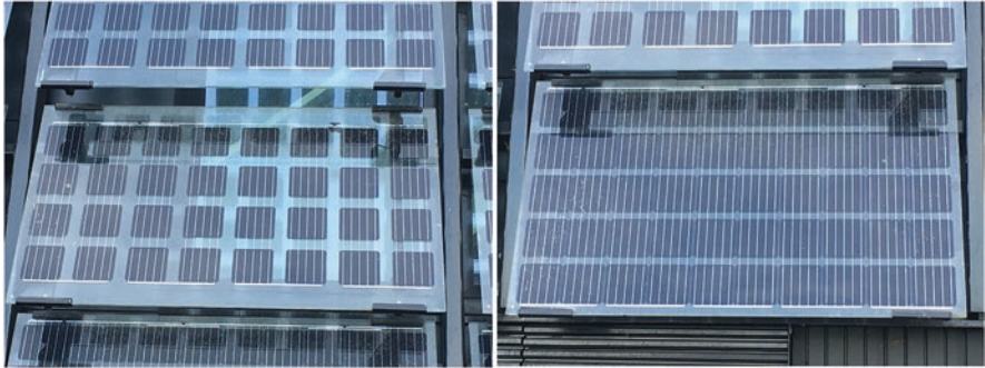
Fig. 22 Different PV panels in the façade with different transparency
