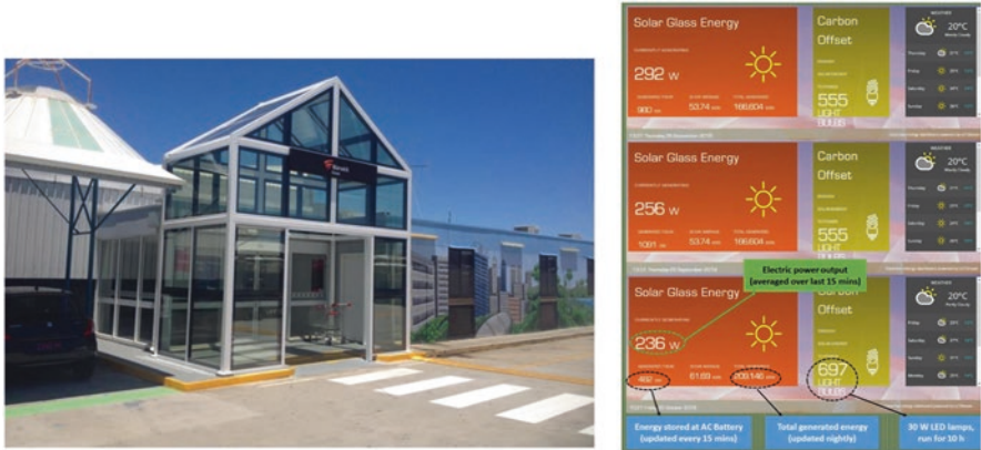
Fig. 6 Warwick Grove Shopping Centre Atrium (Perth, Australia) built using ClearVue solar windows and a summary of measured solar installation performance (18 multi-oriented solar windows in total)
