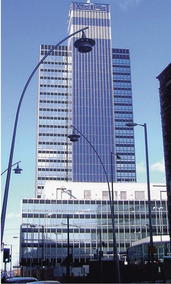
Fig. 4 Building-integrated photovoltaics of the Façade of the CIS Tower in Manchester, England, UK. (Image credit and source: Pit-yacker, https://upload.wikimedia.org/wikipedia/commons/6/6e/CIS_Tower.jpg )
