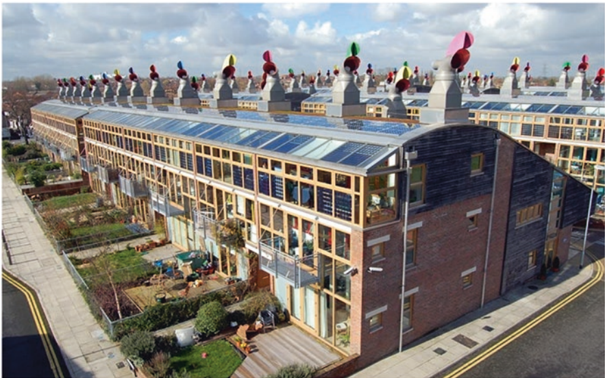
Fig. 25 Mounted solar photovoltaics (PV) on the rooftop of BedZED complex in Beddington, South of London – England, UK. (Image credit and source: Tom Chance, https://upload.wikimedia.org/wikipedia/commons/0/05/BedZED_2007.jpg )
