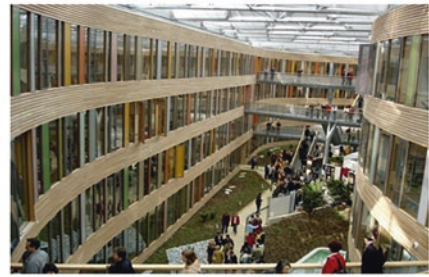
(c) The atrium with the translucent glazed frame holding the solar PV long arrays
