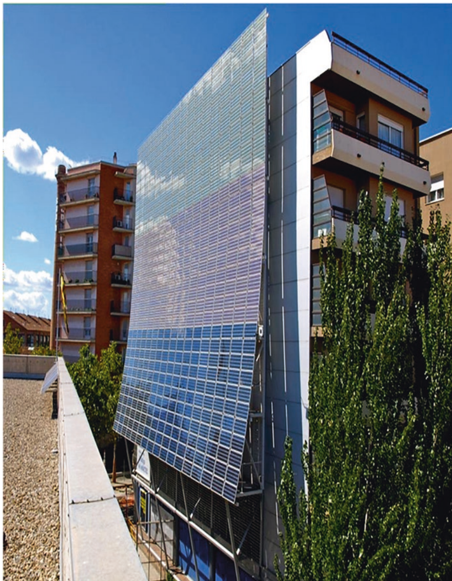
Fig. 3 Building-integrated photovoltaics of the MNACTEC Terrassa in Barcelona, Spain. (Image credit and source: Chixoy, https://upload.wikimedia.org/wikipedia/commons/0/0f/Façana_Fotovoltaica_MNACTEC.JPG )
