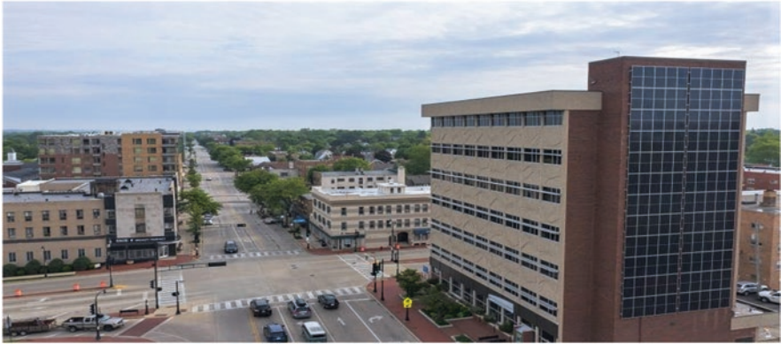
Fig. 3 Office Buildings Complex in Shorewood, WI, USA, more than 25 m high, has “120-module, 54 kW solar array is producing 58,000 kWh annually”. Planned to avoid shading with full safety in mind [6]
