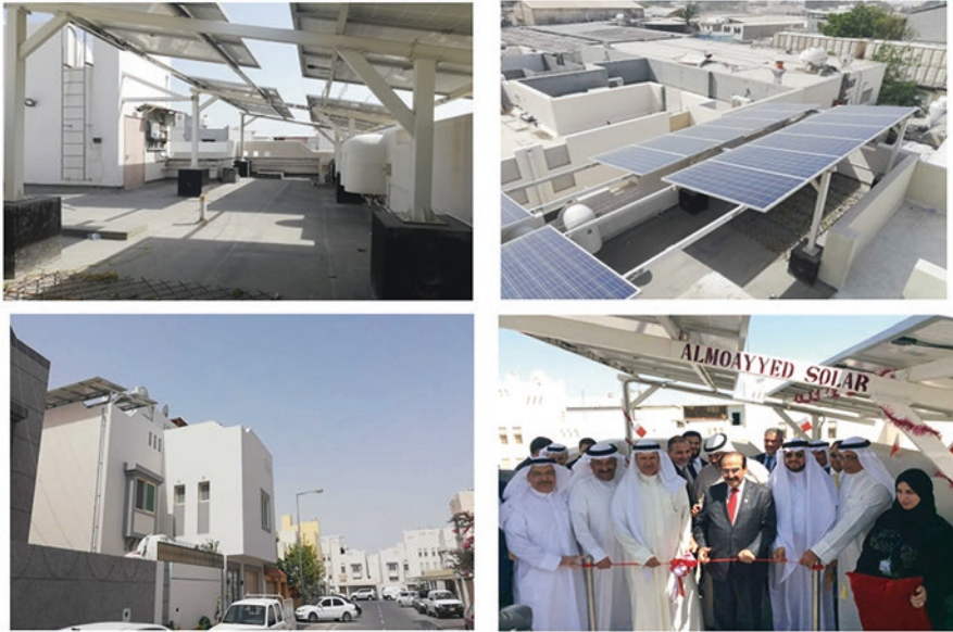
Fig. 48 The layout of the PV panels of the first 7.8 kW PV domestic building (House 4 #108) in Bahrain. Top of PV panels (top right), below the PV panels (top left), during the official inauguration of the project (bottom right) and view of the roof PV from ground (bottom left)
