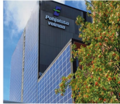
(b) Close up of the BIPV façade of the Toppila power station
