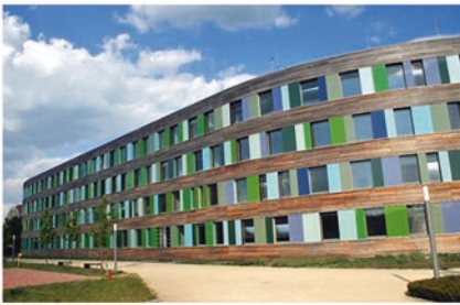
(b) One of the facades of the UBA building, where the solar PV arrays are mounted
