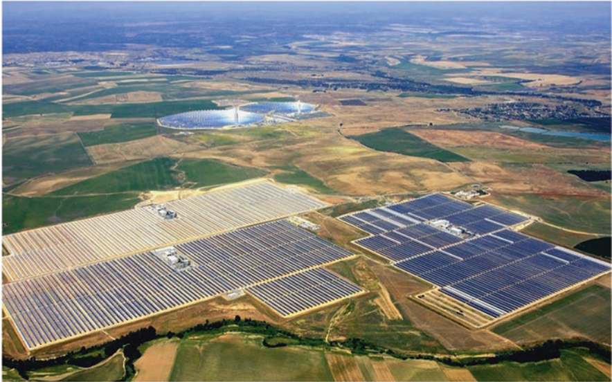
Fig. 32 The first three concentrated solar power (CSP) units of Slovona Power Station in Spain. (Image credit and source: Abengoa Solar, https://upload.wikimedia.org/wikipedia/commons/4/54/Foto_a%C3%A9re_de_Solnovas_y_torre_junio_2010.jpg )
