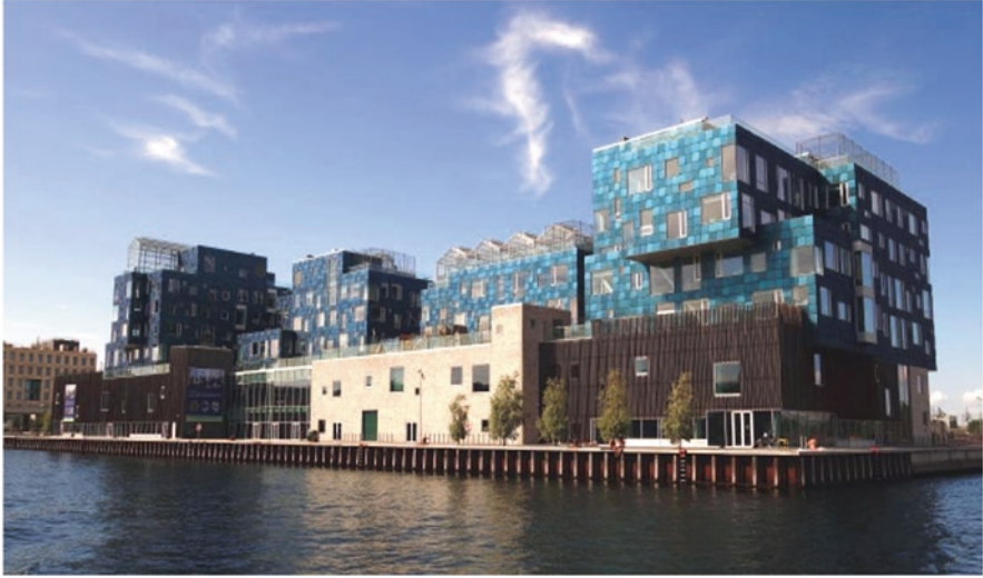
Fig. 11 Back view of the 1200 blue-green colour Photovoltaics façade's panels of Copenhagen International School in Nordhavn, Copenhagen, Denmark. (Image credit and source: MdCAAlmeida Villafuerte, https://upload.wikimedia.org/wikipedia/commons/a/a8/Copenhagen_International_School_-_Nordhavn.jpg )
