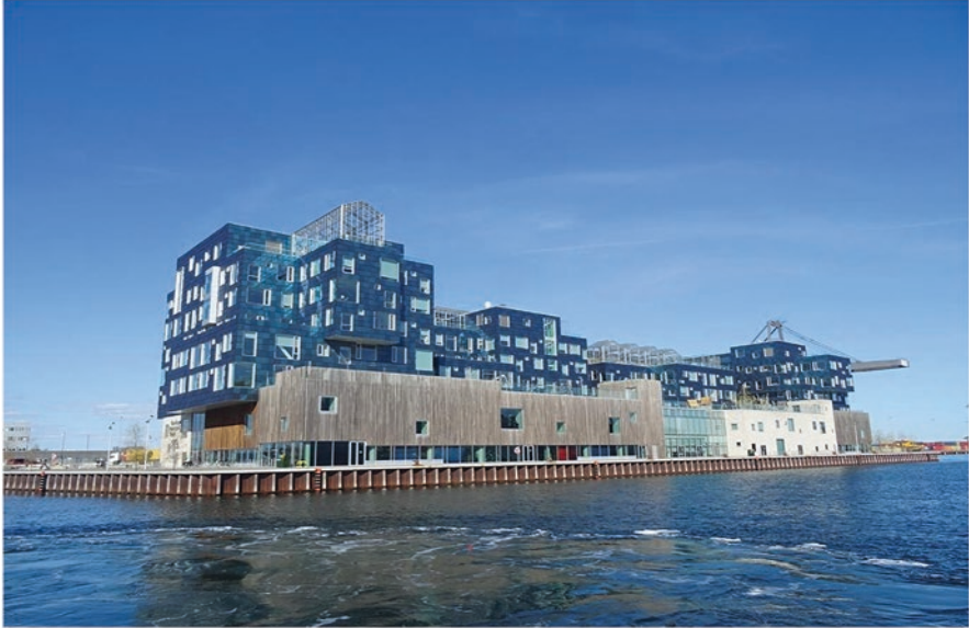
Fig. 12 Close up of the distinctive and eye-catching Copenhagen International School with the blue-green colour Photovoltaics clad all building's facades at Orientbassiniet in Nordhavn, City of Copenhagen, Denmark. (Image credit and source: Leif Jørgensen, https://upload.wikimedia.org/wikipedia/commons/1/1d/Copenhagen_International_School_06.jpg )
