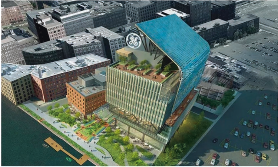
Fig. 13 General view of General Electric New Boston QH featuring ‘Solar photovoltaics veil’ to offset energy cost, Boston, Massachusetts, US. (Image credit and source: General Electric (GE), https://www.treehugger.com/solar-powered-buildings-will-forever-change-architecture-4868157 )
