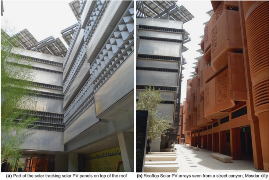
Fig. 24 Close up of building-integrated solar photovoltaics arrays on top of the roofs in Masdar Net-Zero City in Abu Dhabi, UAE. (Image credit and source: (a) and (b) Mohsen Aboulnaga) (a) Part of the solar tracking solar PV panels on top of the roof. (b) Rooftop Solar PV arrays seen from a street canyon, Masdar city
