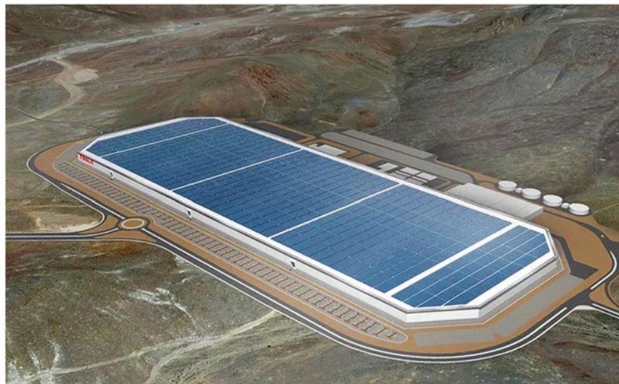
Fig. 26 An impression of Tesla's Net-zero Gigafactory powered by huge roof-mounted PV arrays in Nevada, USA, the largest building by physical areas worldwide and powered by renewable sources. (Image credit and source: Tesla, https://www.treehugger.com/solar-powered-buildings-will-forever-change-architecture-4868157 )
