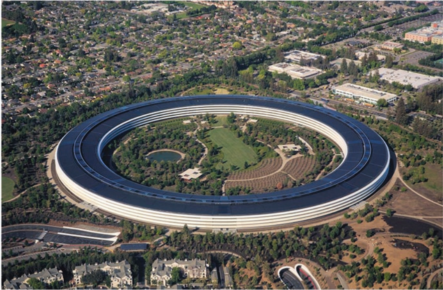
Fig. 7 Building-integrated solar photovoltaics panels generate 17 MW power at Apple Park, the corporate headquarters of Apple Inc., in Cupertino – California, USA. (Image credit and source: Daniel L. Lu (user: Dllu), https://upload.wikimedia.org/wikipedia/commons/5/5a/Aerial_view_of_Apple_Park_dllu.jpg )
