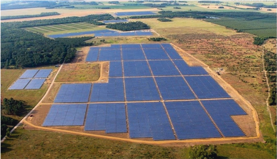
Fig. 30 Jännersdorf solar park generating clean power in Prignitz, Germany. (Image credit and source: Parabel GmbH, https://upload.wikimedia.org/wikipedia/commons/4/48/Solarpark_Jännersdorf.jpg )
