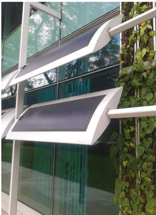
Fig. 29 Solar PV external shading devices in a zero-energy building in Singapore, Singapore. (Image credit and source: Esmail7, https://www.wikiwand.com/en/Photovoltaic_mounting_system )
