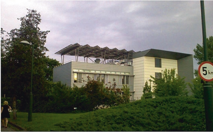
(a) Main façade of the REC Conference Centre with mounted 140 solar PV array on its roof
