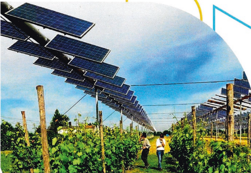
Fig. 4 The use of PV for agriculture, project AIAS, an EU project representing different countries [7]
