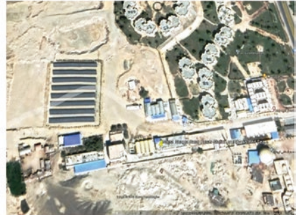
(b) Aerial view for Marsa Shagra Power Station, Red Sea, to be expanded (Image Source: Authors via Google Earth)
