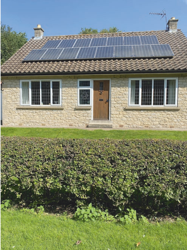
Fig. 1 A typical home development, in the UK with PV installation.
