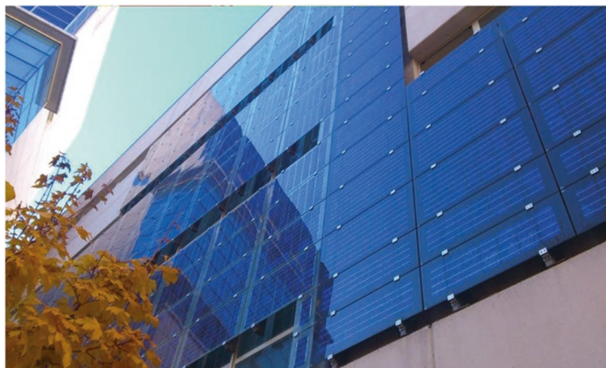
Fig. 1 Integrated solar photovoltaic façade of the municipal building, social services, Centre Jose Villarreal in Madrid, Spain. (Image credit and source: Hanjin, https://upload.wikimedia.org/wikipedia/commons/f/f8/BAPV_solar-facade.JPG )
