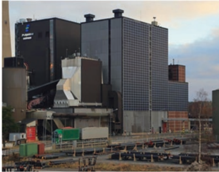
(a) General view of the Toppila power plant showing the BIVP on the southern façades
