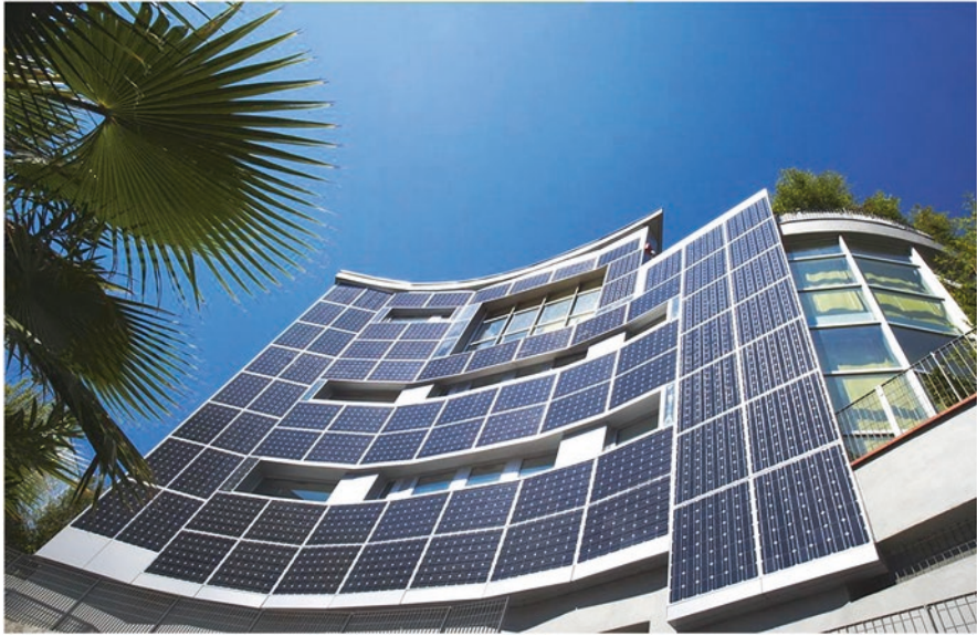
Fig. 17 A set of integrated solar PV arrays on the front façade of a residential building in Singapore, Singapore. (Image credit: https://www.yoursunyourenergy.com/upload , source: https://energypedia.info/wiki/File:BIPV.jpg#/media/File:BIPV.jpg )
