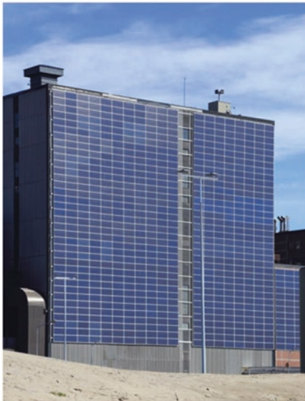
(c) Building-integrated photovoltaics of the southern façade of the Toppila power plant generating clean energy
