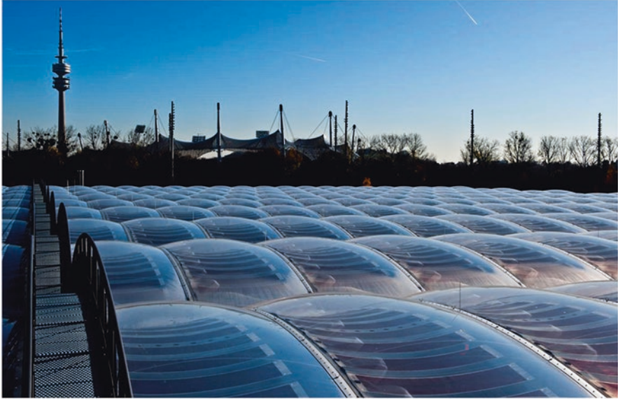
Fig. 8 ETFE Cushions' roof with integrated Photovoltaics of the AWM Munich's Municipal Waste Management Department in Munich, Germany. (Image credit and source: MdCALmeida Villafuerte, https://upload.wikimedia.org/wikipedia/commons/a/ac/AWM-Munich-ETFE-Cushions-Photovoltaics.jpg )
