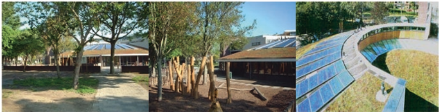
Fig. 10 First Dutch NZEB school with its BIPV
