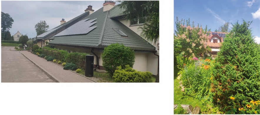
Fig. 6 Examples of micro PV systems installed on a roof of a single-family house (right) and small hotel (left)
