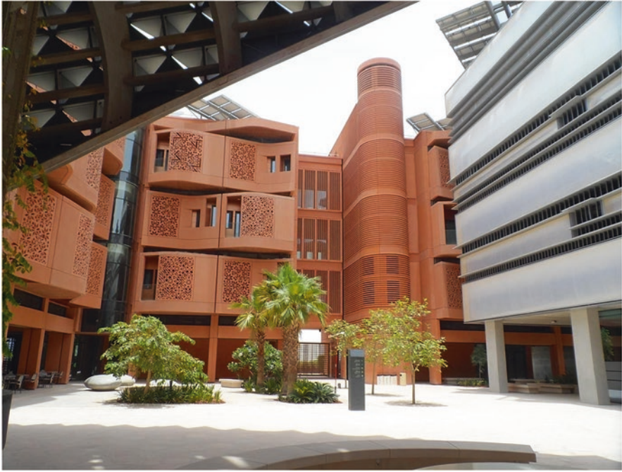
Fig. 22 Integrated solar photovoltaics arrays on top of buildings' roofs in Masdar City in Abu Dhabi, UAE. (Image credit and source: Mohsen Aboulnaga)
