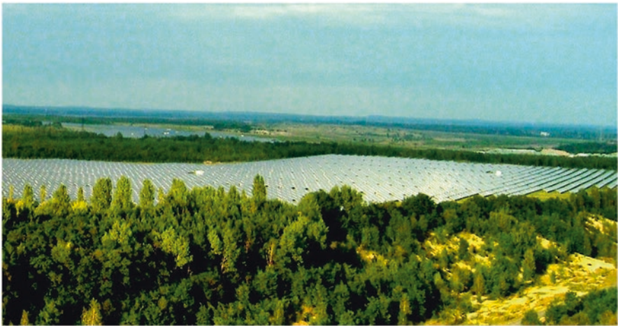
Fig. 33 Part of the Senftenberg 78 MW Solar Park located in the former open-pit mining areas near the city of Senftenberg, Eastern Germany. (Image credit and source: Z Thomas, https://upload.wikimedia.org/wikipedia/commons/4/45/Blick_vom_aussichtsturm_H%C3%B6rlitz4.jpg )
