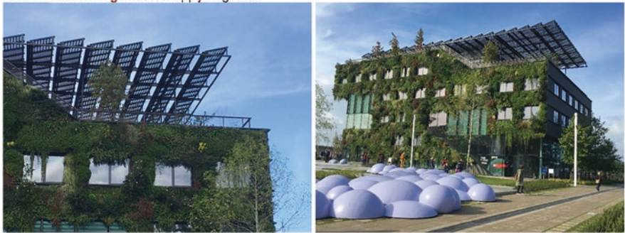
Fig. 25 The 'tropical roof' of Ares Hogeschool
