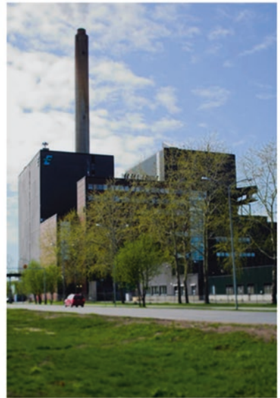
(d) The site of the Toppila power station where the Solar PV array is installed on its façades
