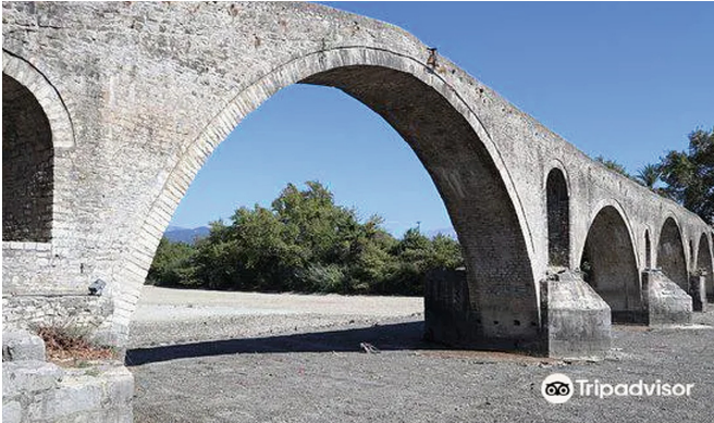
Fig. 2. The Bridge of Arta [Source: youimg1.tripcdn.com]
