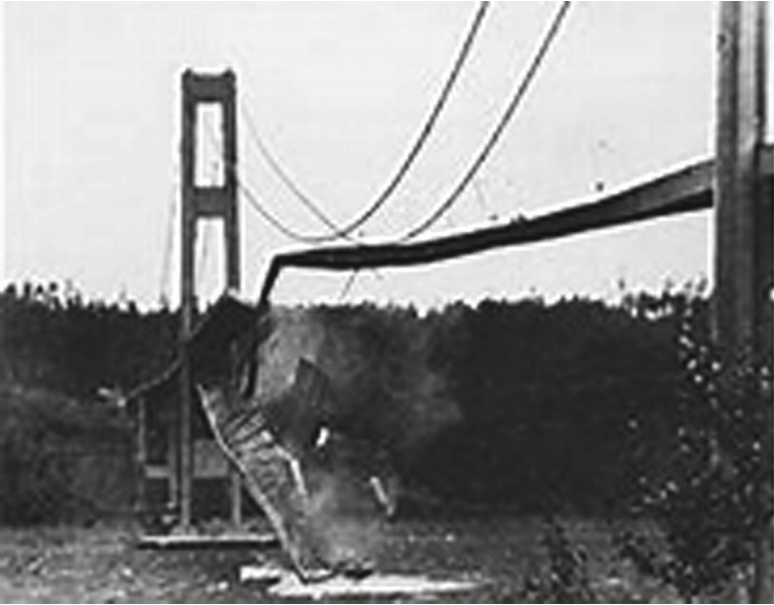
Fig. 3. The collapsed Tacoma Bridge
