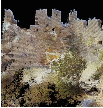
Fig. 9. The exterior east side of Palaiokastro Gate, registered point cloud from Magnet Collage.
