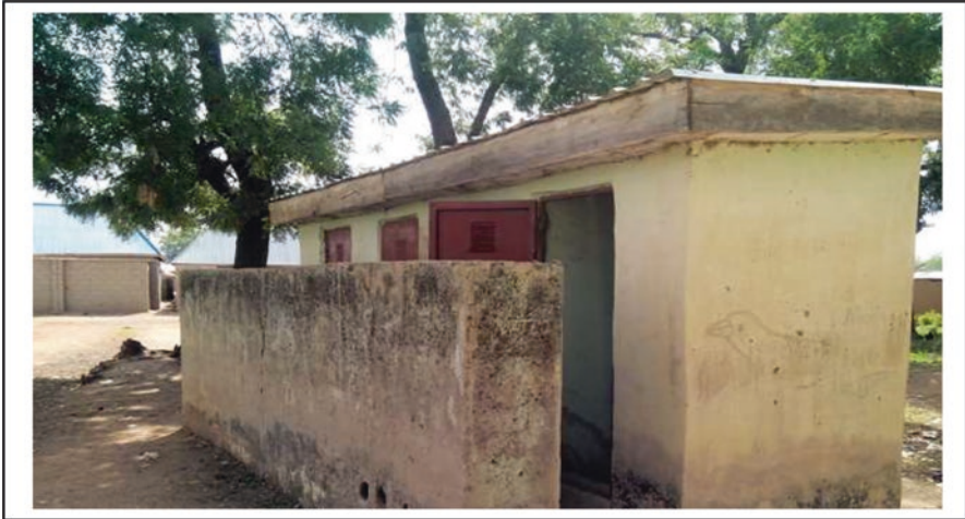
Fig. 14.18 Another toilet facility in one of the schools in Bauchi state
