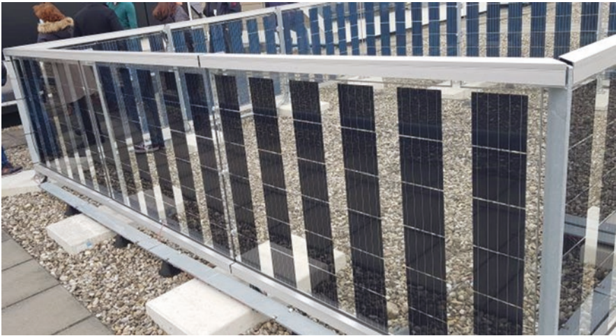
Fig. 4.15 Experimental semitransparent balcony – Eindhoven University. (Photographer Cotfas Daniel Tudor)
