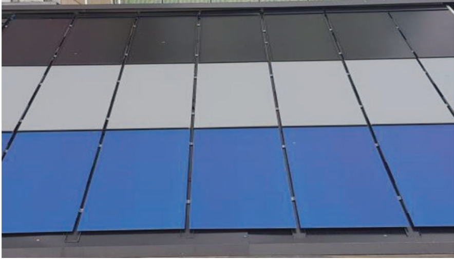
Fig. 4.11 Experimental colored photovoltaic panels – Eindhoven University. (Photographer Cotfas Daniel Tudor)
