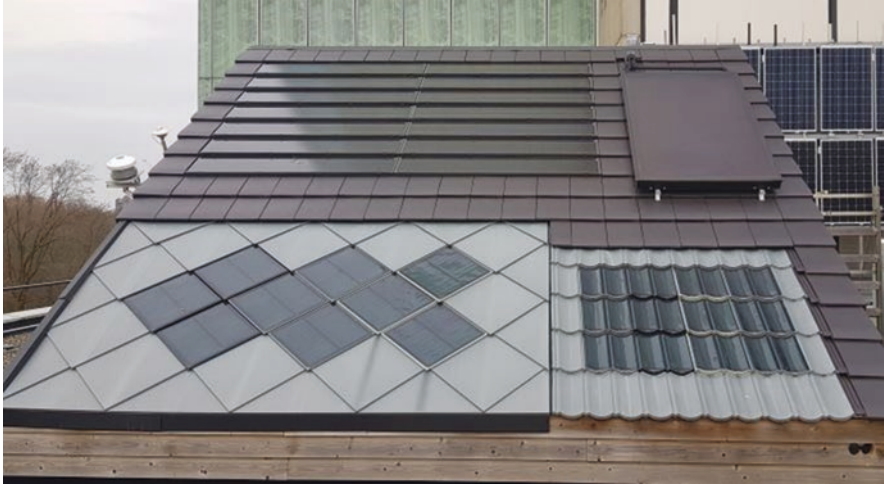
Fig. 4.9 Experimental photovoltaic panels with tiles – Eindhoven University. (Photographer Cotfas Daniel Tudor)
