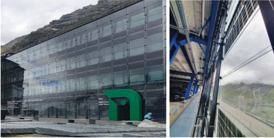
Fig. 4.14 Semitransparent façade – Parkhaus Gletscherbahn at Kaiser Franz Josefs Höhe. (Photographer Cotfas Petru Adrian)
