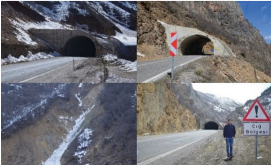
Fig. 11.2 Avalanche tunnels and “avalanche zone” warning sign on Erzincan-Tunceli motorway
