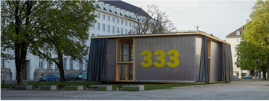
Fig. 3 Pavillon 333 has been realised as a DesignBuild project at the TUM Department of Architecture, next to the Pinakothek der Moderne in Munich, as a temporary and collaboratively used mediation space for architecture, art and design. The Pavillon promotes cooperation between the local cultural institutions and offers low-threshold services, exchange and encounters for visitors to the Munich art area. Photo by Matthias Kestel for TUM, 2022
