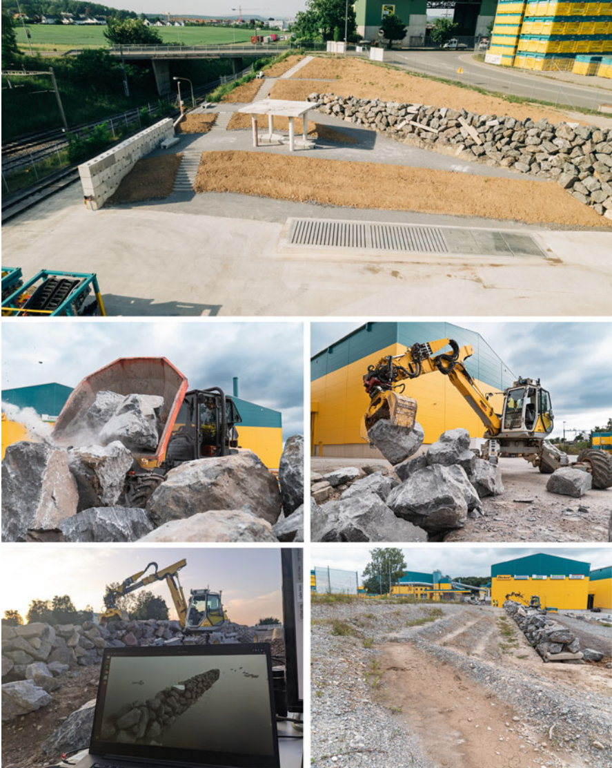
Fig. 9.2 (i) The Circularity Park is a full-scale and publicly accessible landscape park built with robotic landscaping and autonomous robotic dry-stone masonry, utilising HEAP. The material includes locally sourced boulders and waste concrete (ii). The main enabling technologies facilitating the on-site adaptive construction process included (iii) an adaptive planning computational design and tool and (iv) a scanning process for digitising the individual stones. Robotic landscaping enabled precise landscaping of the surrounding terraces (v). (© Gramazio Kohler Research. Drone Videography: Girts Apskalns. Photography: Mark Schneider)
