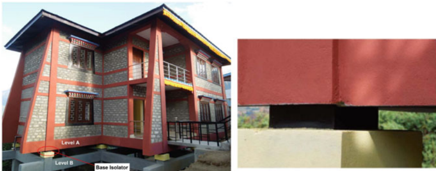
Fig. 3 Base-isolated masonry building located in Tawang, India (Thuyet et al.)
