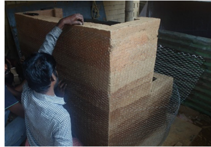
Fig. 2. Reinforcement with wire mesh.
