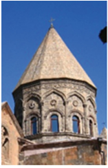
Fig. 15. Dome and drum
