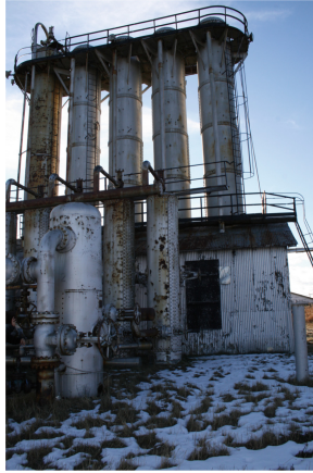
Fig. 1. The absorption building at the Turner Valley Gas Plant.
