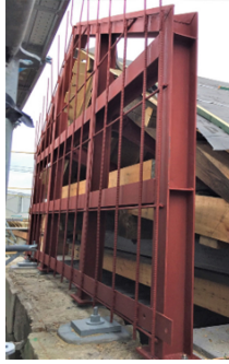
Fig. 13. Reinforcement of pediment by steel frame
