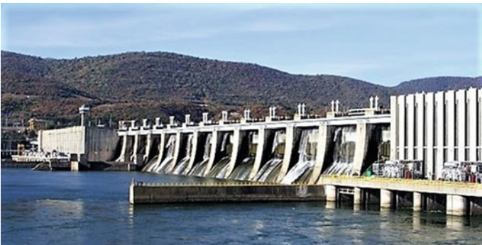
Fig. 13.102 Iron gates I dam and hydropower plant
