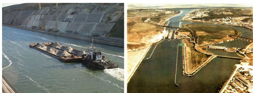
Fig. 13.104 The Danube-Black Sea canal (left) and Agigea hydrotechnical node (right)
