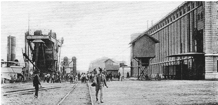
Fig. 13.15 Reinforced concrete silos, port of Brăila
