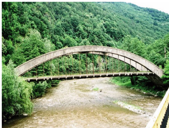
Fig. 13.43 The bridge at Lainici
