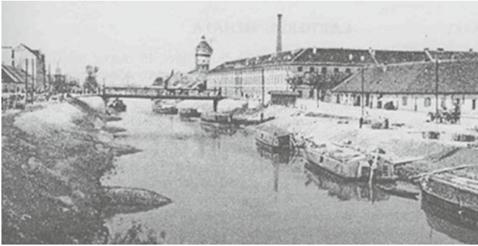
Fig. 13.45 Port of Timisoara on the Bega Canal
