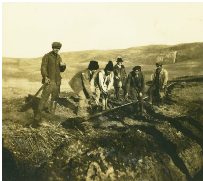
Fig. 6 The construction of transport pipes in Transylvania
