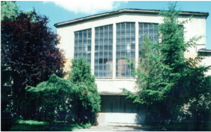
Fig. 3 The Hydraulic Machines Laboratory of Timișoara, 1953
