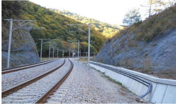
Fig. 13.118 Rehabilitated sector on the railway Bucharest—Predeal between Comarnic and Valea Largă
