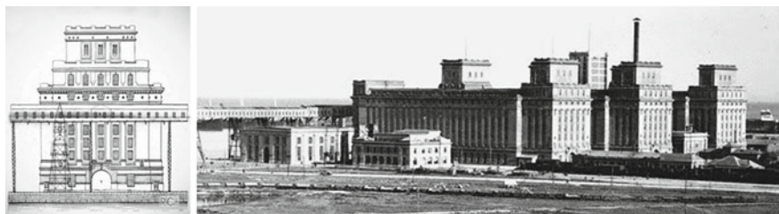
Fig. 13.47 Silos in Constanța port: drawing for one unit (left) and overview (right)
