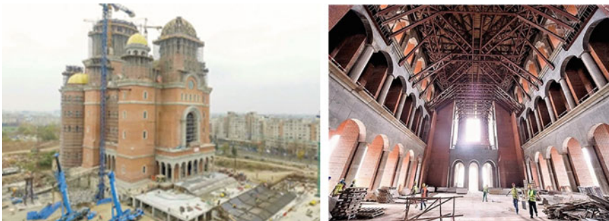
Fig. 13.112 Cathedral during construction
