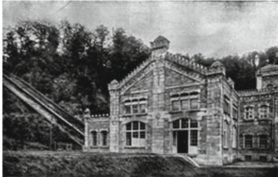
Fig. 13.48 The hydropower plant Grebla
