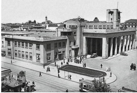
Fig. 13.56 Bucharest North railway station, main entrance with the monumental portico
