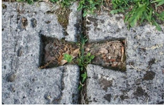
Fig. 13.2 Murus dacicus, stone block assembly system
