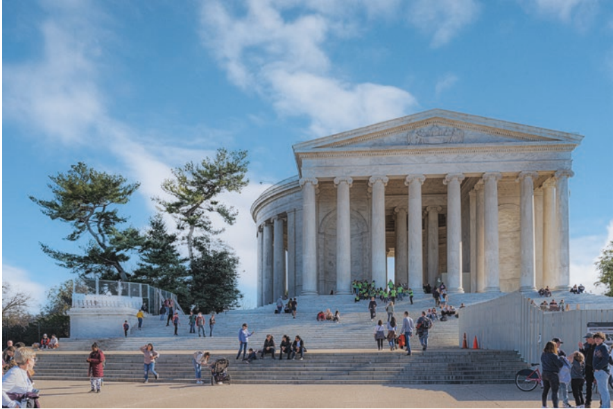
Fig. 6.2 The Jefferson Memorial is a beautiful structure done in the classical style. Handrails are not apparent, but the building is being renovated. Photo by Stephen Fadem
