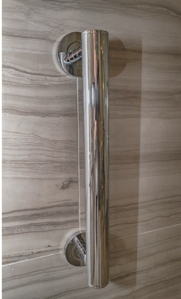
Fig. 3.4 The loss of balance is a major reason for falling. Using a grab bar can prevent a serious injury
