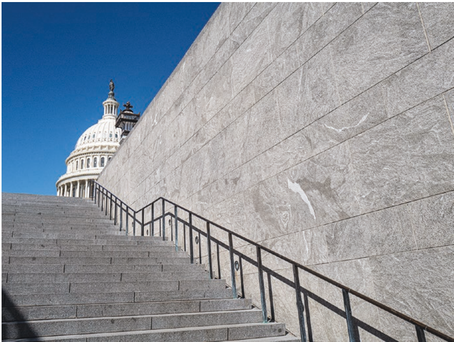
Fig. 6.1 Handrails prevent falls. Trying to walk on the stairs while holding objects and not holding on to the rails is a fall risk, particularly in the elderly. Photo by Stephen Fadem
