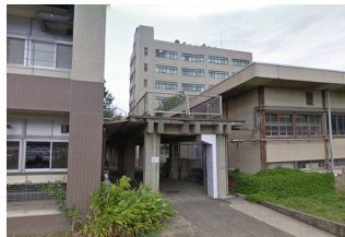
Fig. 3. Bridge site and structure.
