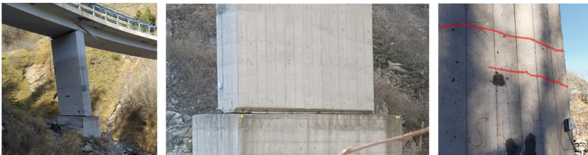
Fig. 2. View of the current configuration of pillar 1.
