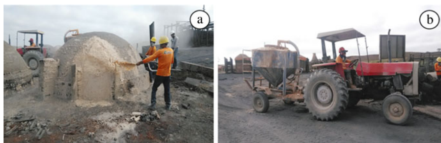
Fig. 3 Cooling of the kilns through the application of water and clay (a) with the aid of a tractor, Massey Ferguson 275 model (b) (Source The authors 2023)
