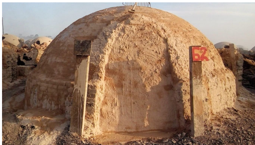
Fig. 2 Rudimentary brick kiln commonly used in charcoal production with SFMP wastes in Brazilian Amazonia (Source The authors 2023)
