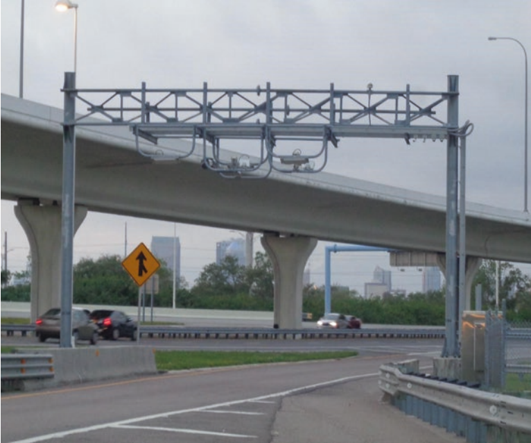
Fig. 6.1 Toll gantry for toll-by-plate payments, Selmon Expressway
