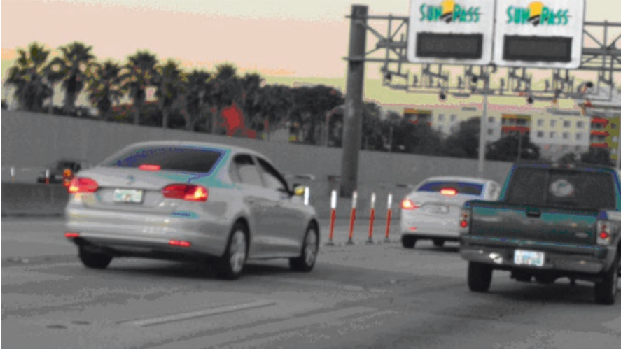
Fig. 3.4 Overhead toll gantry with RFID wireless system
