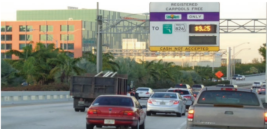
Fig. 3.6 Dade County, FL I-95 North HOT lane (peak hour)
