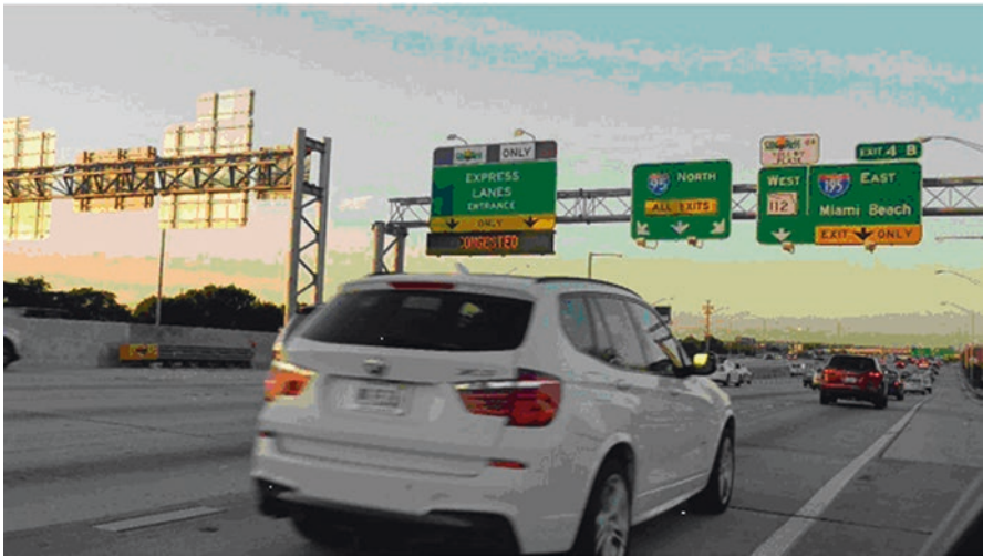
Fig. 3.8 I-95 Express lane entrance (Miami-Dade, FL)
