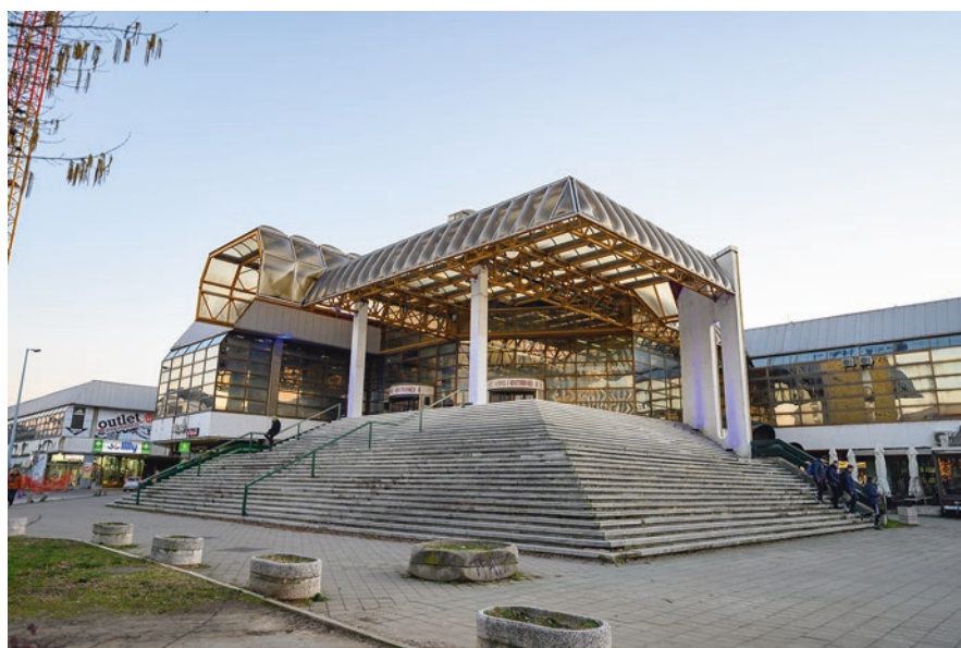
Fig. 3 Spens—the Sports and Business Centre of Vojvodina, exterior. Photo by Igor Đokić; © 2022 by BAZA—Spatial Praxis Platform
